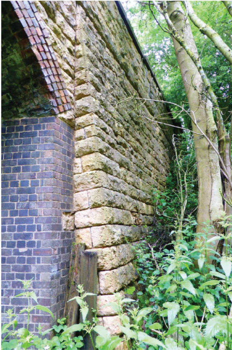
13) North east wingwall
