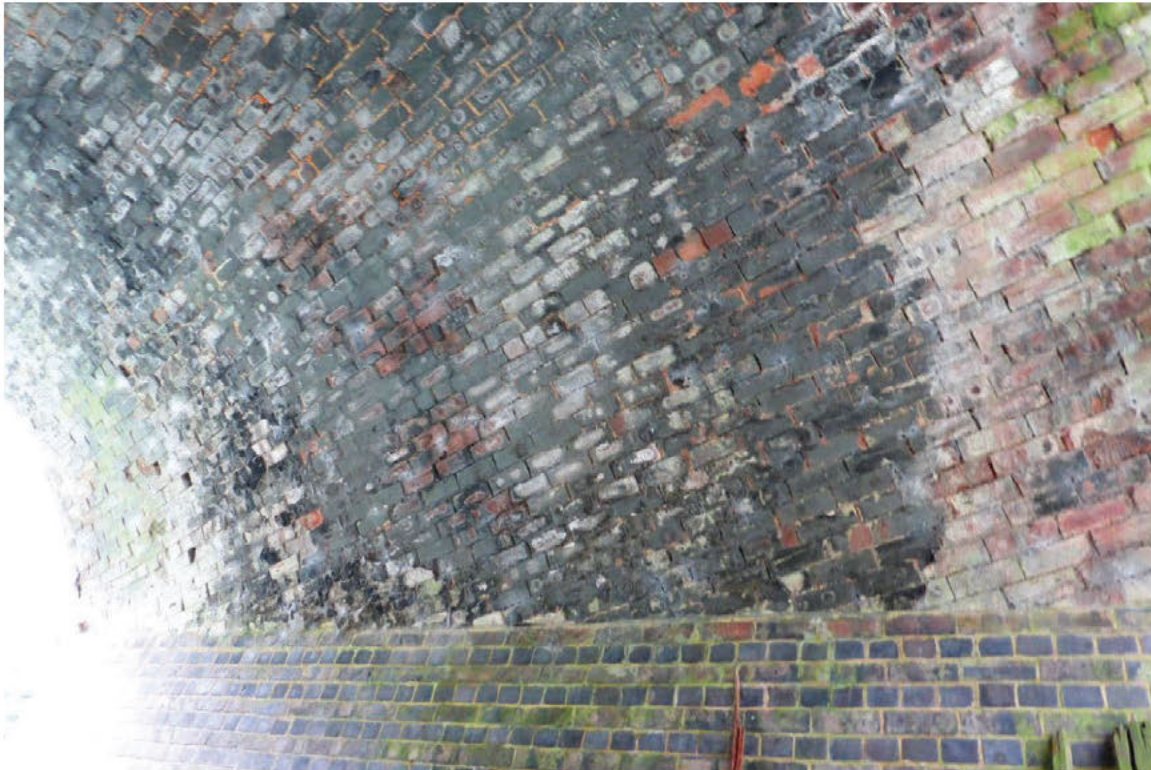
7) South east view of the arch barrel
