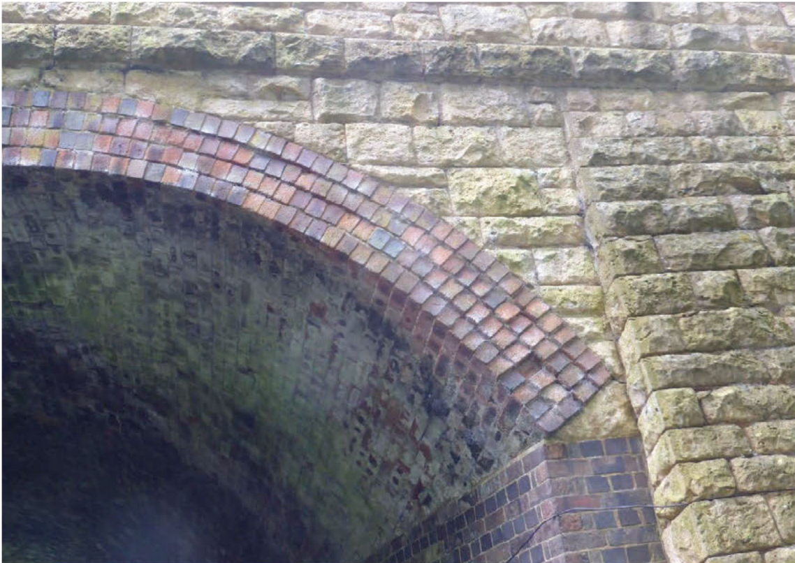
17) South west spandrel
