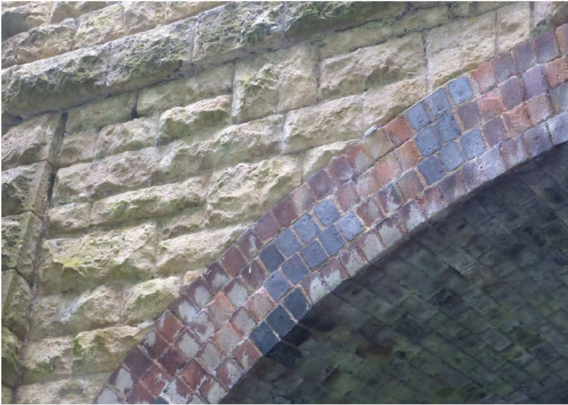
16) North west spandrel
