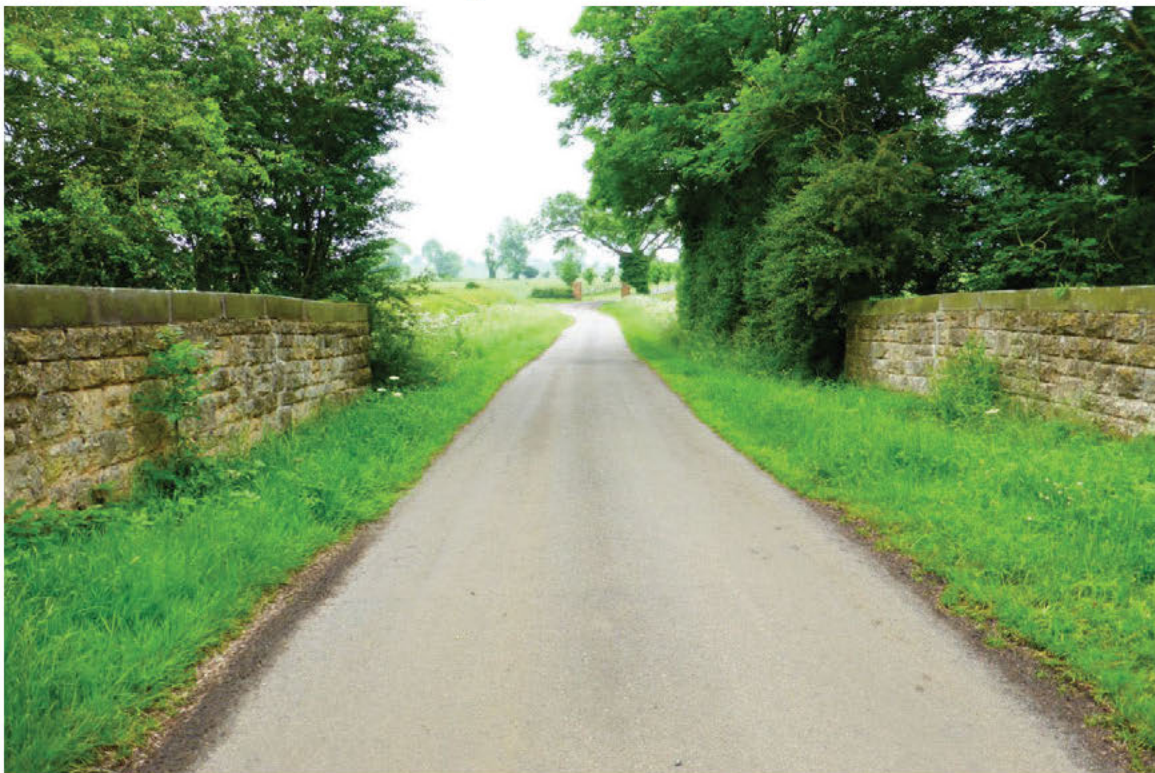
4) View of carriageway approach looking south
