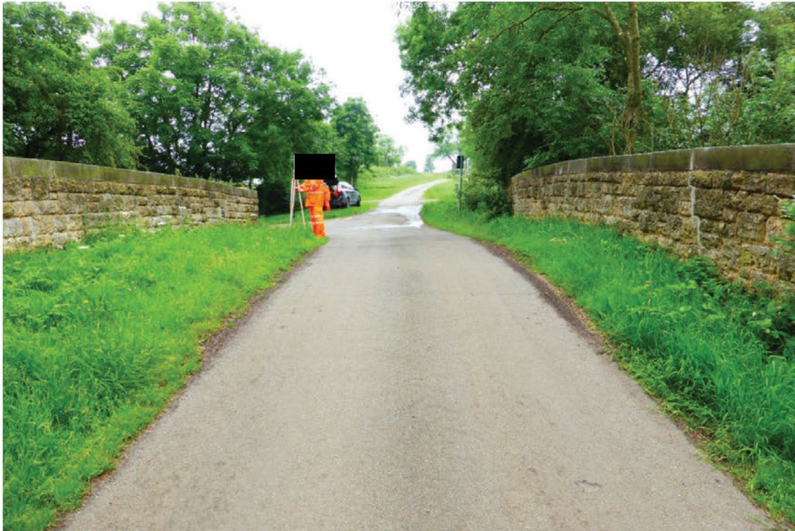
3) View of carriageway approach looking north
