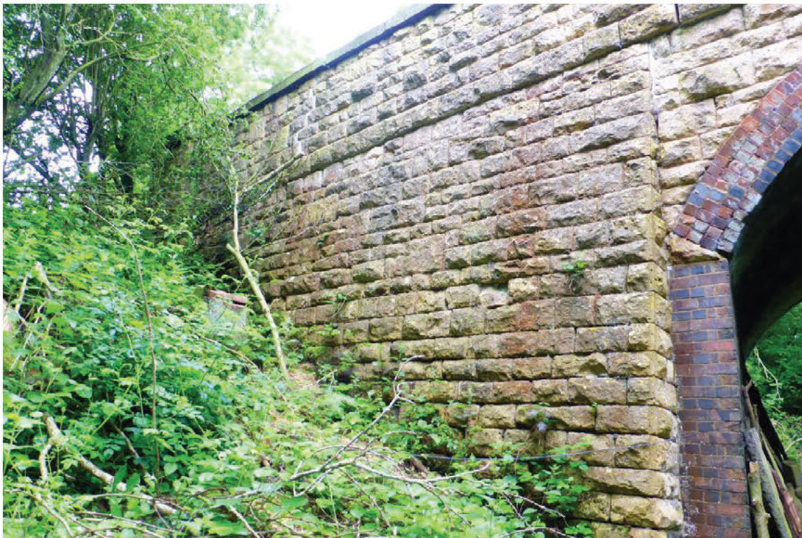
12) South east wingwall
