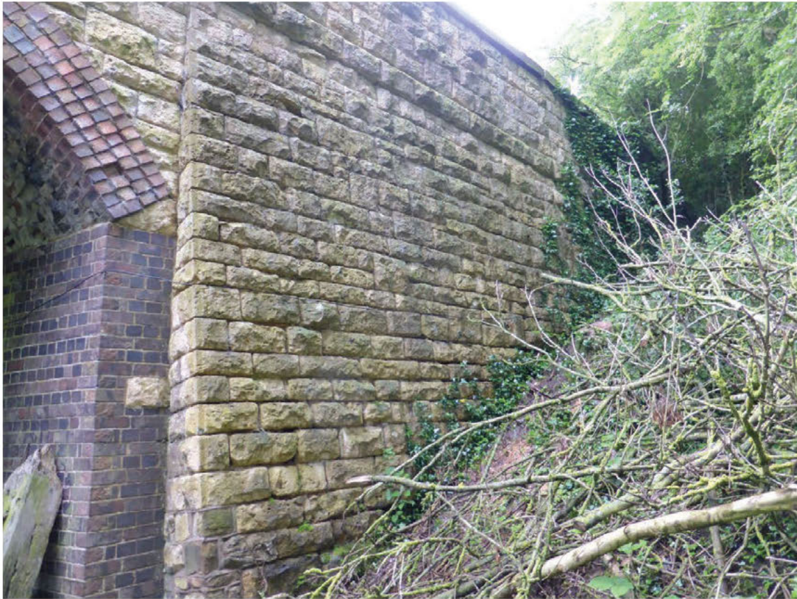
14) South west wingwall
