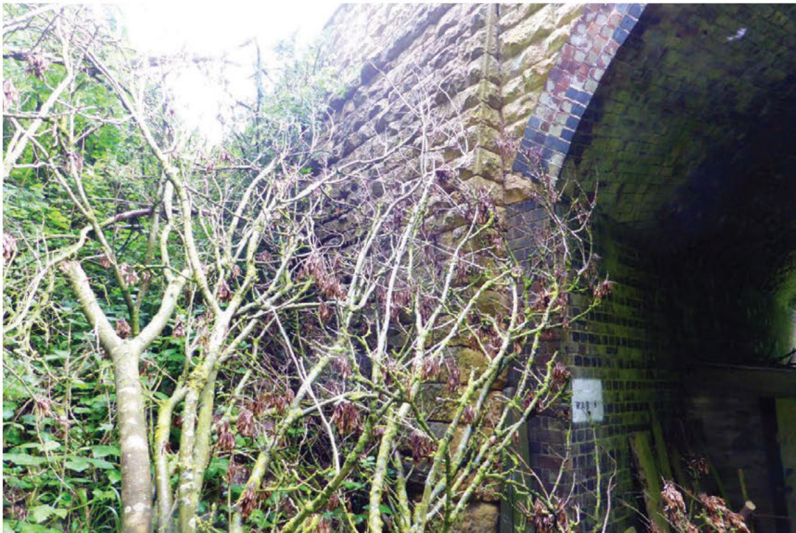
15) North west wingwall
