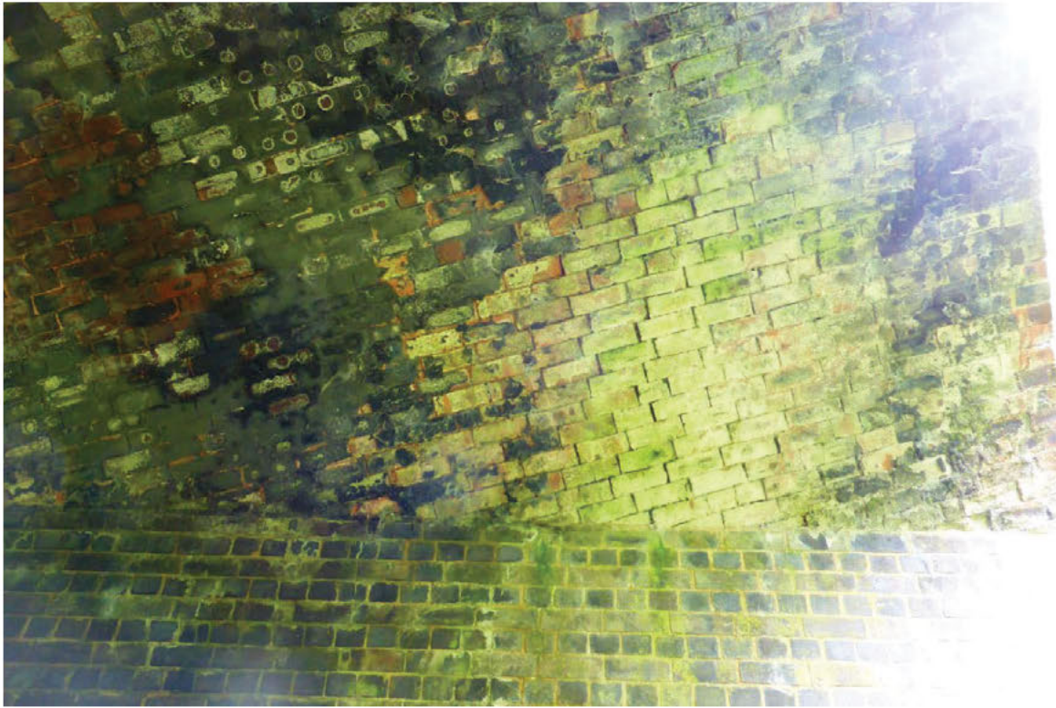
5) North east view of the arch barrel
