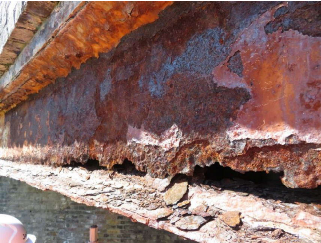
Photograph 16. South Edge Girder at Midspan – External face and web
