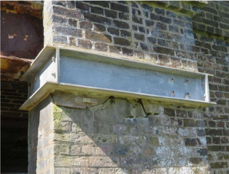
Photograph 37. Southeast wingwall - buttress
