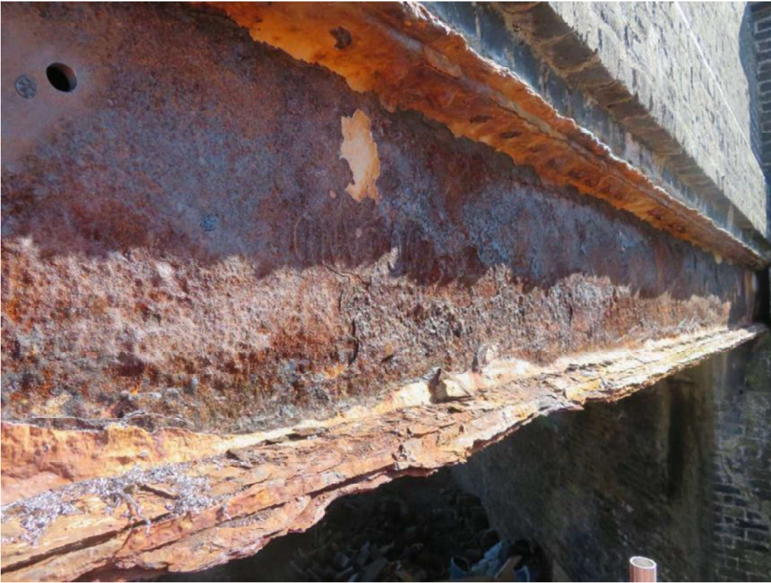
Photograph 21. North Edge Girder at Midspan – External face and web
