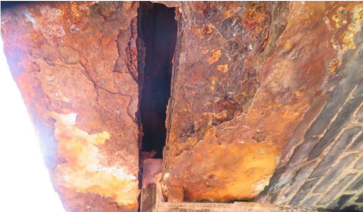
Photograph 17. South Edge Girder at Midspan – Underside of Bottom Flange
