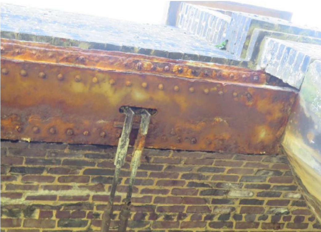
Photograph 20. North Edge Girder at East Support – Underside of bottom flange plate
