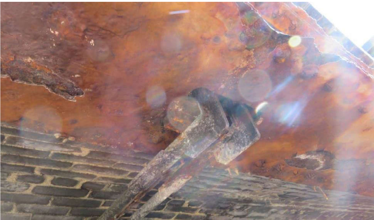
Photograph 22. North Edge Girder at Midspan – Underside of Bottom Flange
