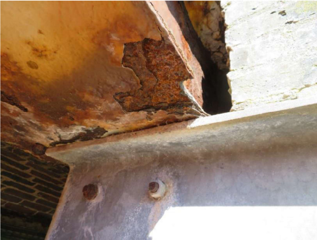
Photograph 15. South Edge Girder at East Support – Underside of bottom flange plate
