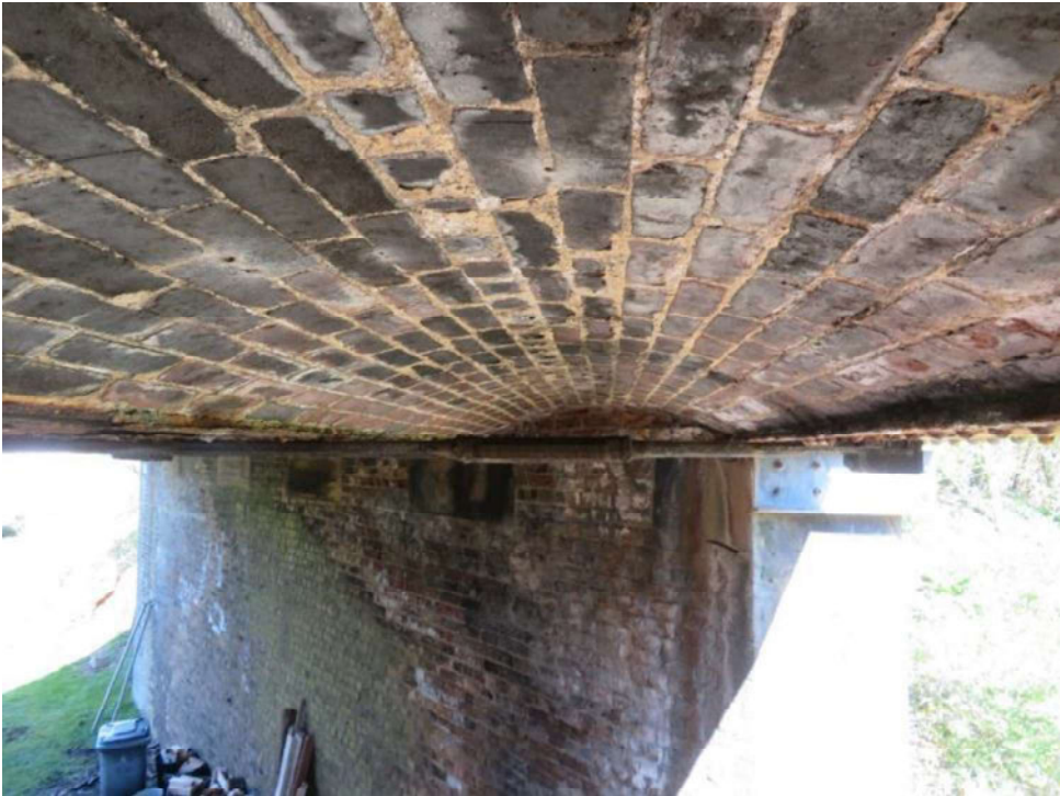
Photograph 7. Soffit (View South along east edge girder)
