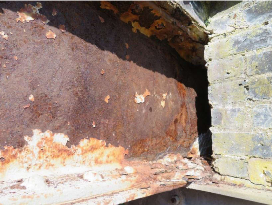
Photograph 19. North Edge Girder at East Support - Web
