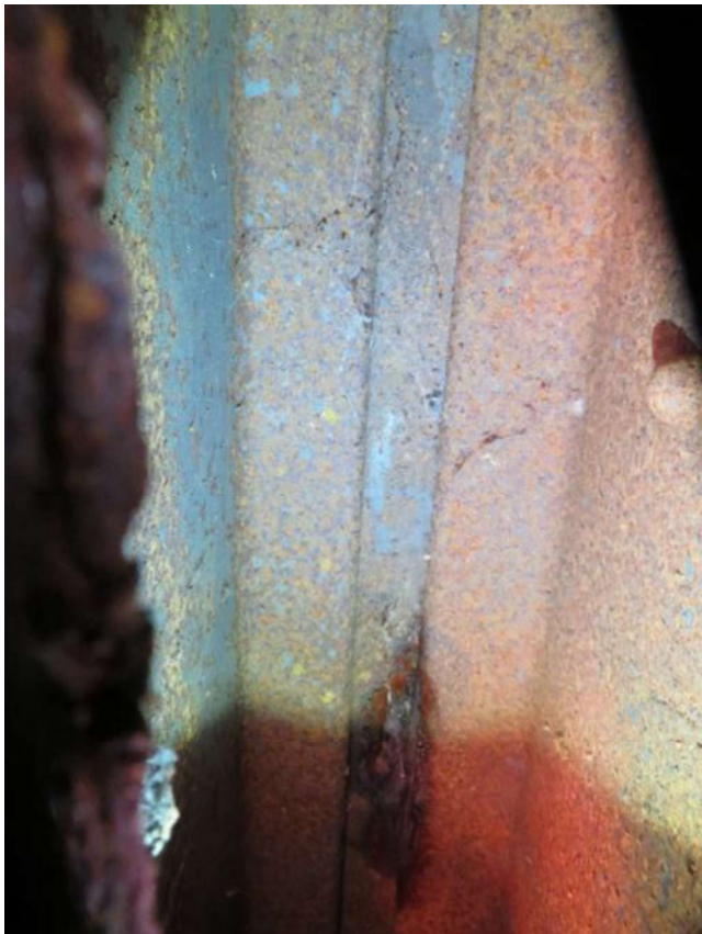
Photograph 18. South Edge Girder at Midspan – Internal Faces
