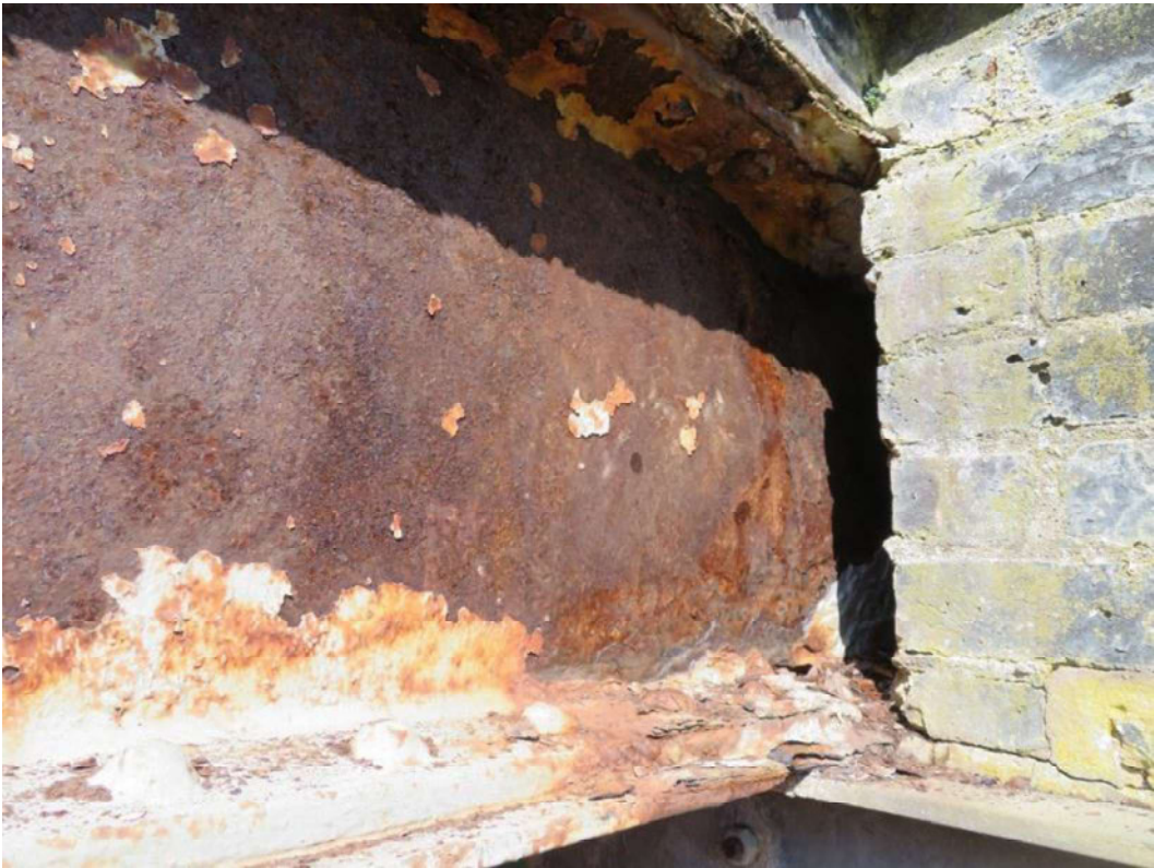
Photograph 14. South Edge Girder at East Support - Web
