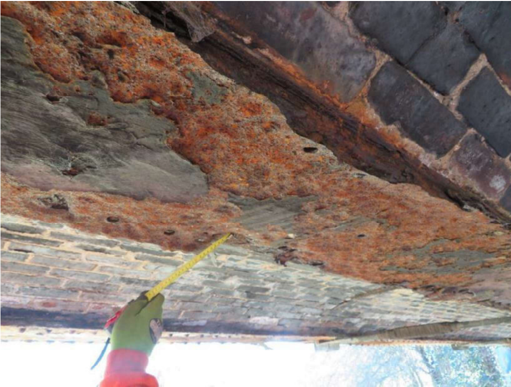
Photograph 25. Second Internal Girder from South - Midspan
