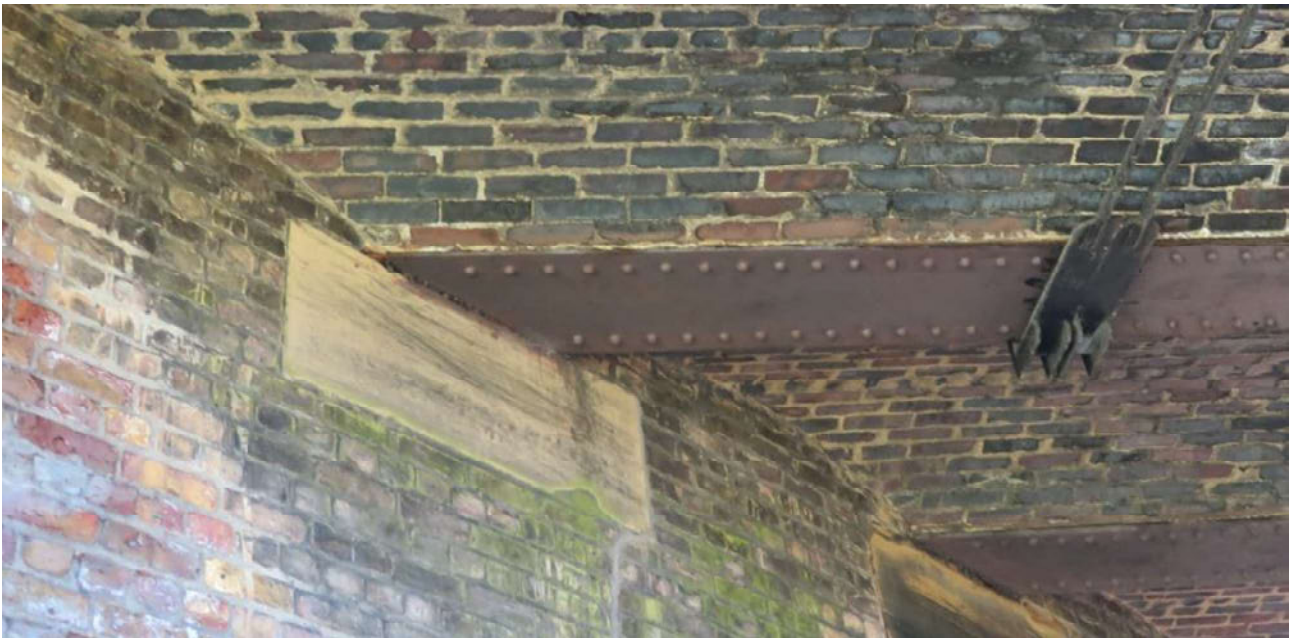
Photograph 24. Second Internal Girder from South - Support
