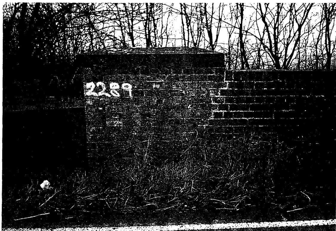
F31/10 - Vertical crack between old and newer brickwork on east parapet
