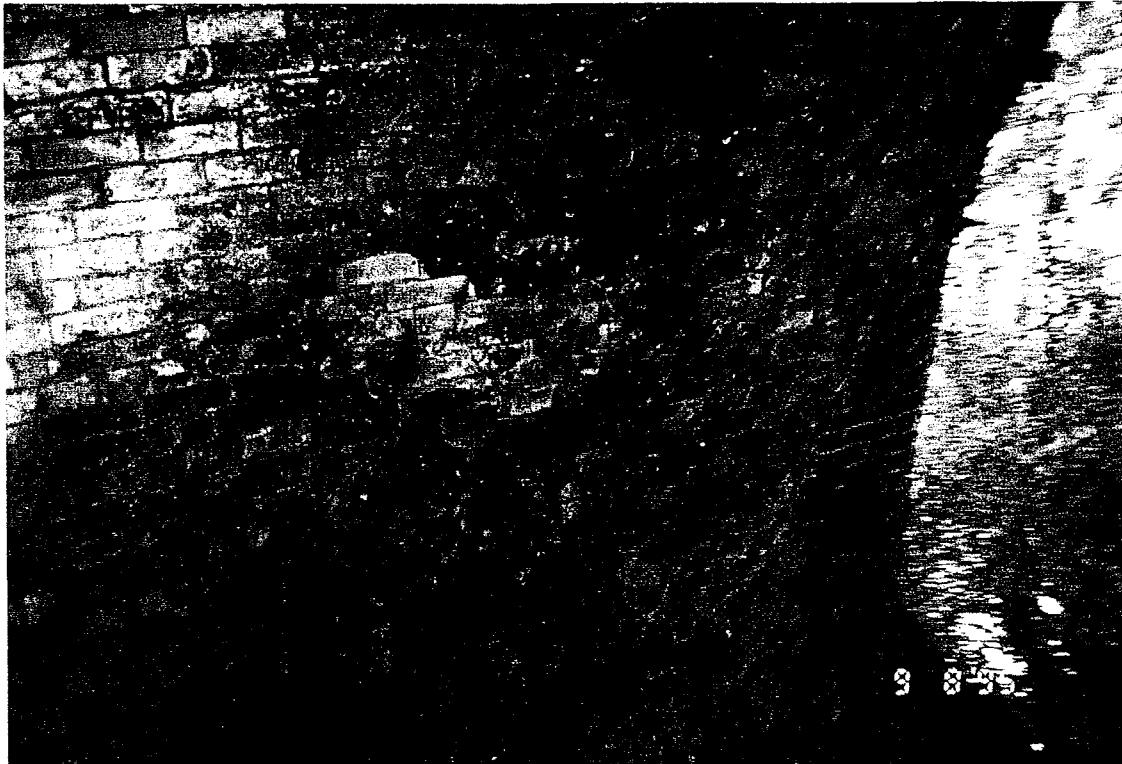
F14/11 - Spalling along the east edge of the barrel.
