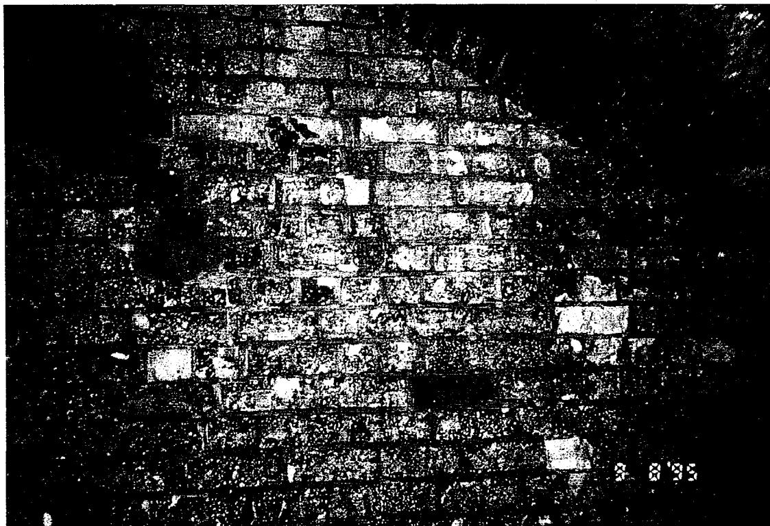
F14/5 - Efflorescence in the centre of south west wingwall.
