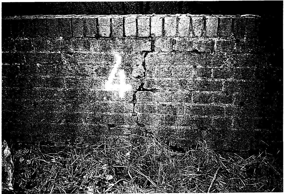
F31/2 - Vertical crack in west parapet
