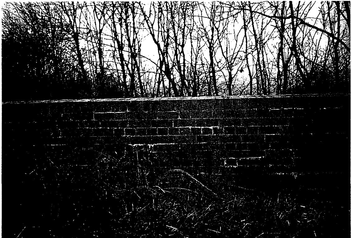
F31/12A - Hairline cracks with efflorescence in east parapet
