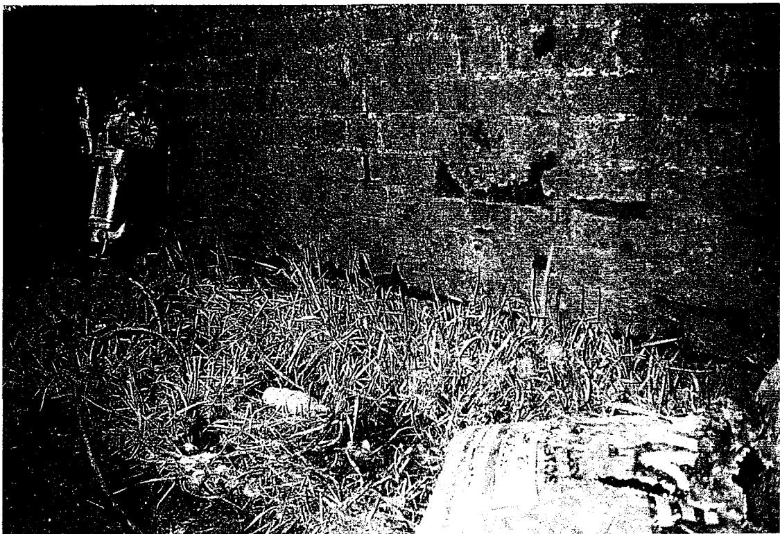
F31/3 - Mortar loss along base of west parapet
