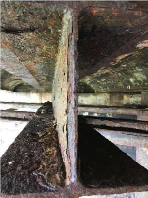
Photograph 37 - Worst propping beam beneath 1 st internal girder from south web reduced to 5mm at top and 3mm at bottom
