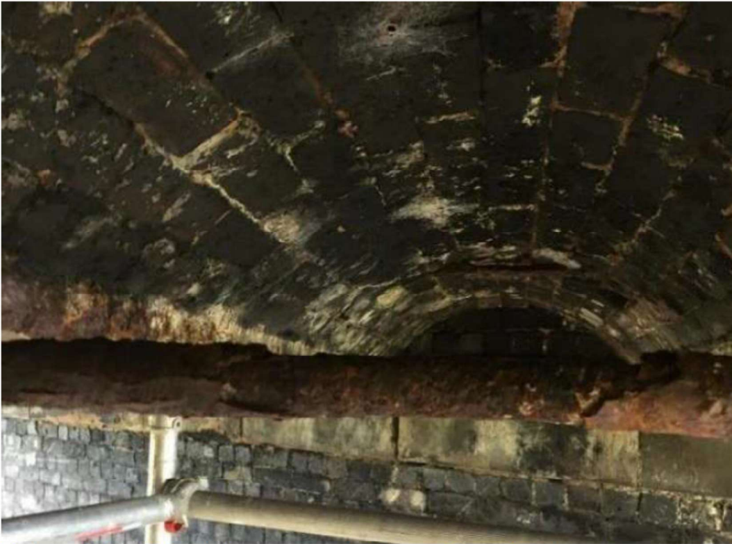
Photograph 31 - New tie bars are corroded down to 25mm diameter
