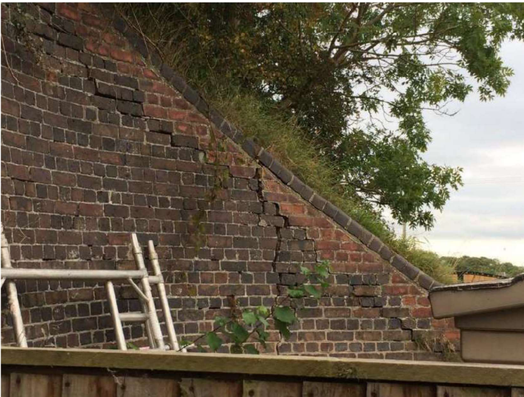
Photograph 34 - Section of south east wingwall separated away for 50mm at a vertical crack
