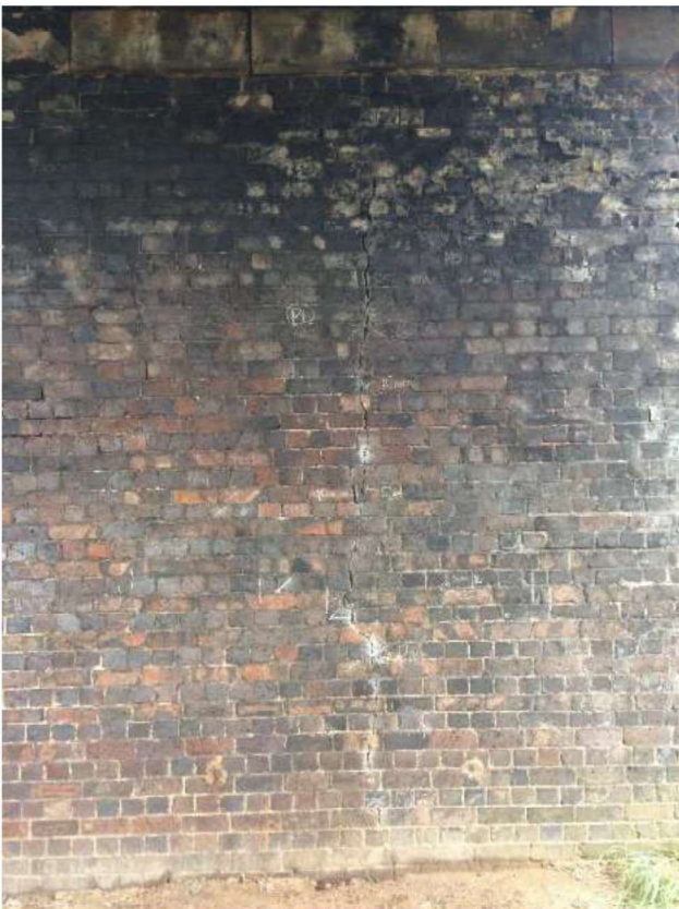
Photograph 32 - Full height vertical crack to east abutment up to 10mm wide.
