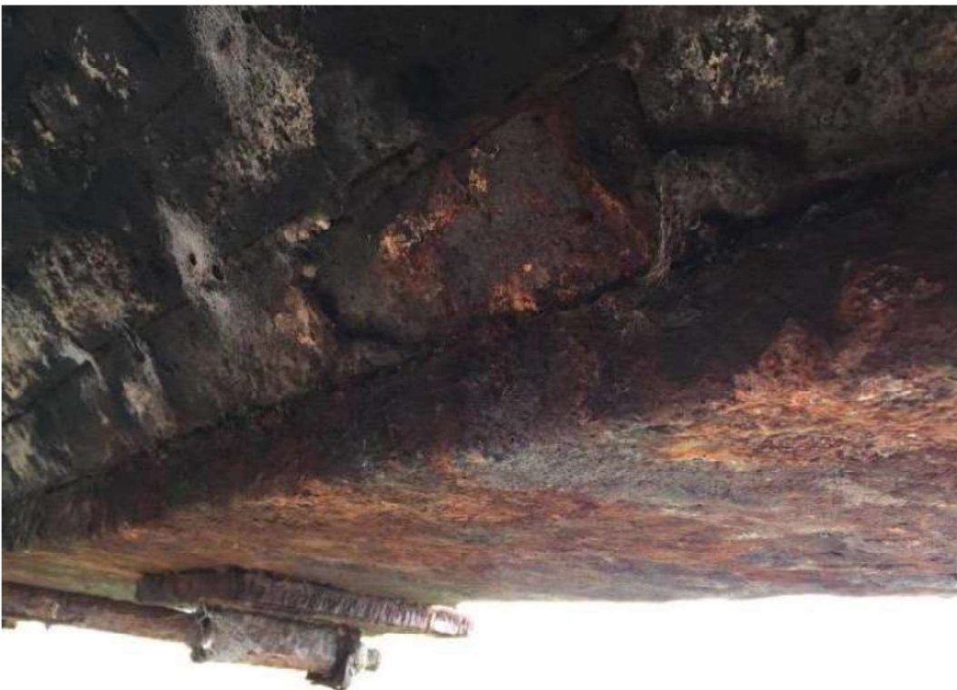
Photograph 24 - North edge girder bottom flange delamination typically 1mm deep, up to 3mm deep over historic blast zones.
