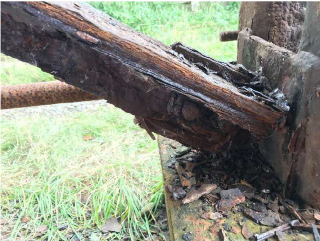
Photograph 40 - Corrosion to angle bracing with worst case showing 5mm thickness remaining
