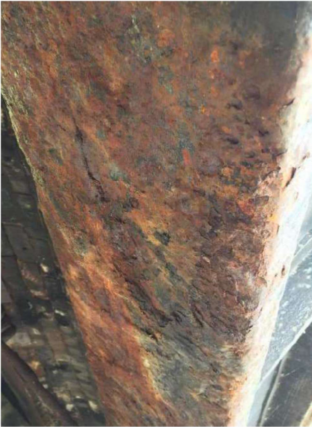
Photograph 21 - South edge girder exhibits delamination to bottom flange.
