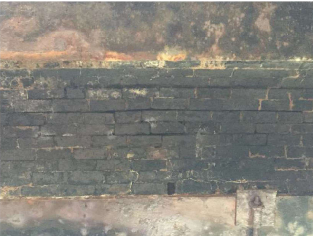
Photograph 28 - Five bricks dropped by up to 30mm with extensive mortar loss to crown of central jack arch.
