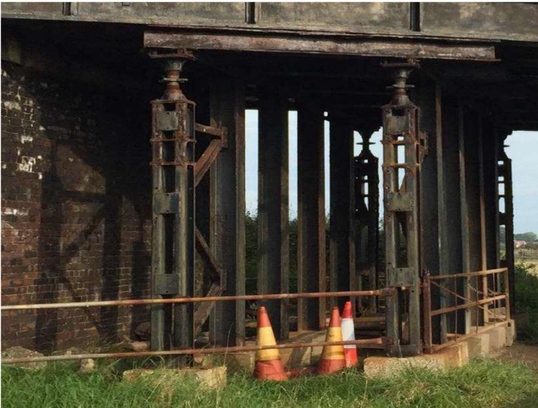
Photograph 9 - General view of propping system
