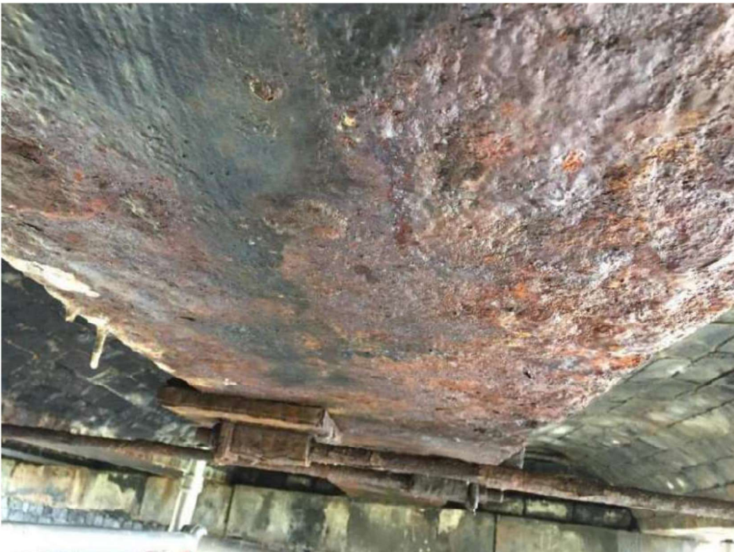
Photograph 26 - Corrosion to bottom flange of first internal girder from the south.
