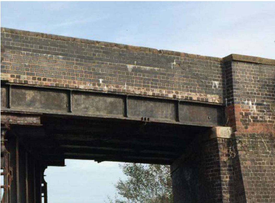
Photograph 35 - Diagonal crack to west end of south parapet outer face.
