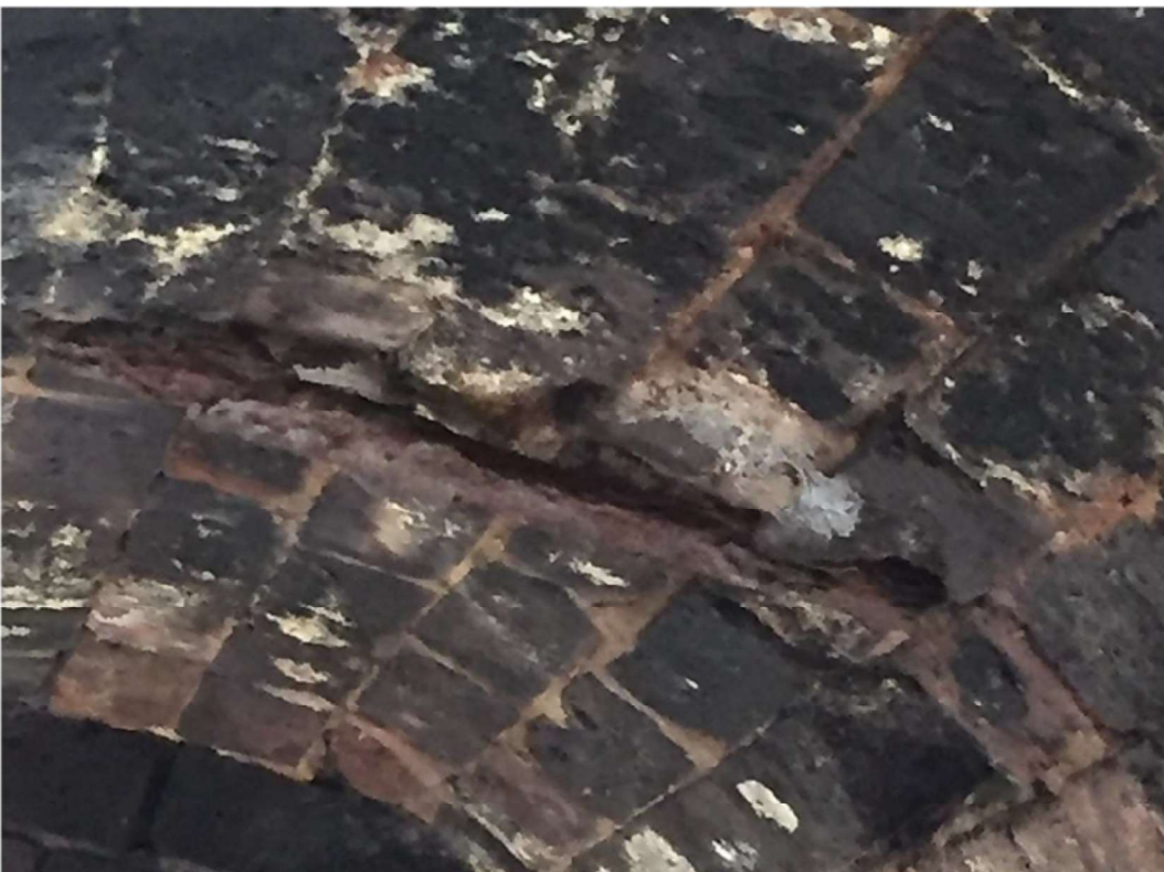
Photograph 30 - Original tie bars severely corroded
