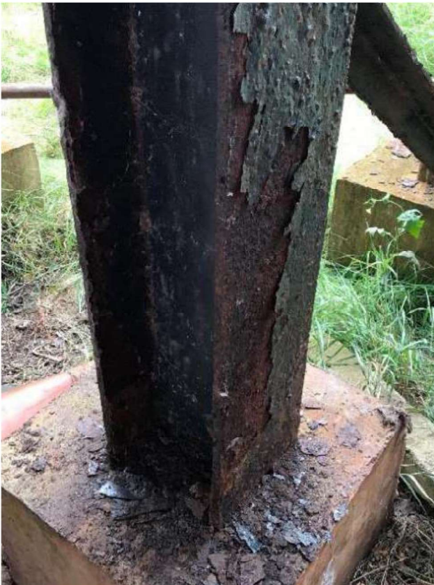
Photograph 38 - Internal columns are typically delaminated up to 1mm deep.
