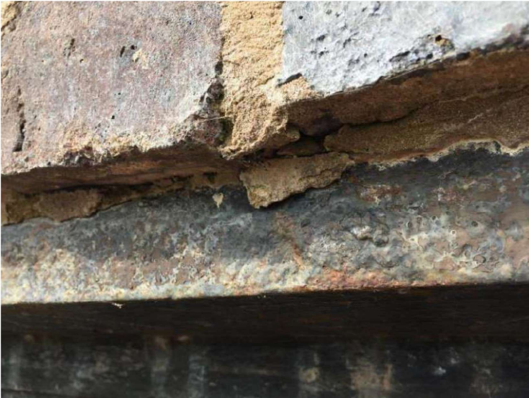
Photograph 23 - South edge girder top flange edge shows pitting along entire length up to 2m deep
