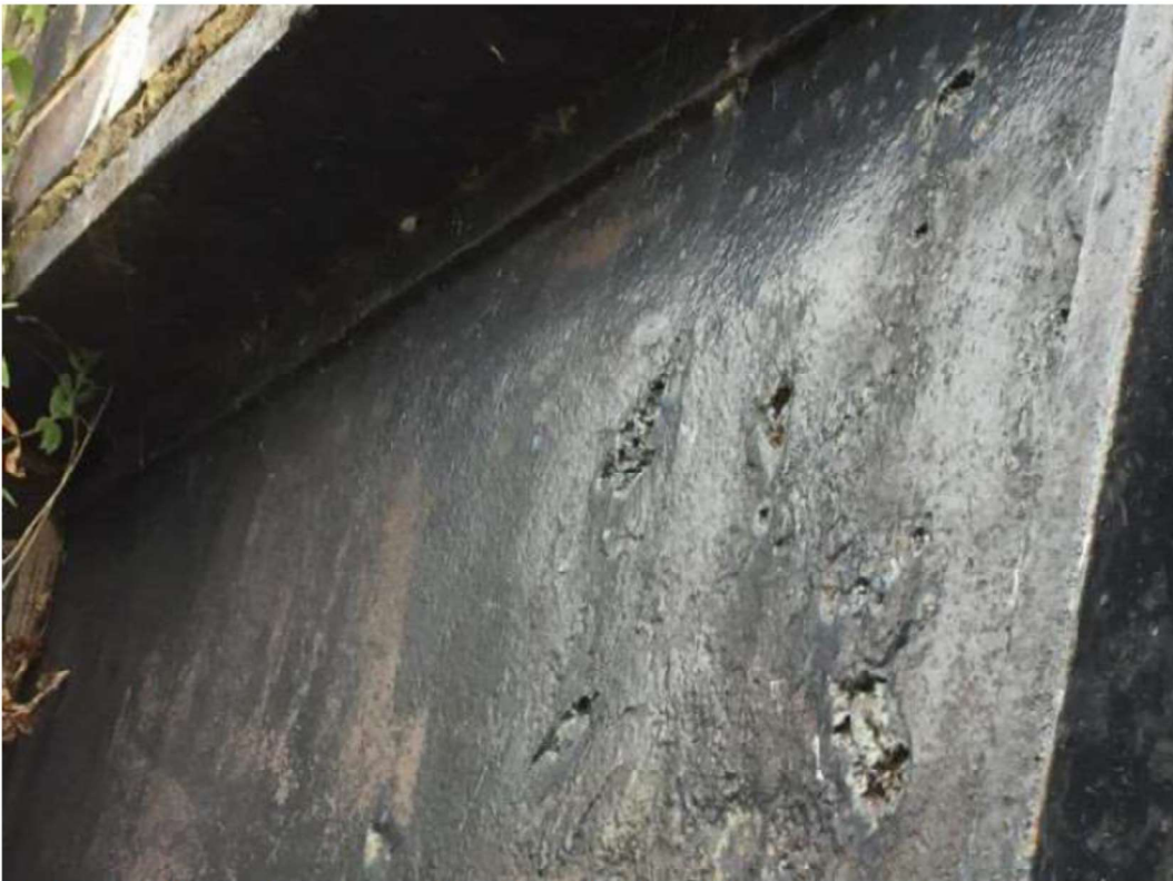
Photograph 25 - Corrosion patches to north edge girder web up to 5mm deep.
