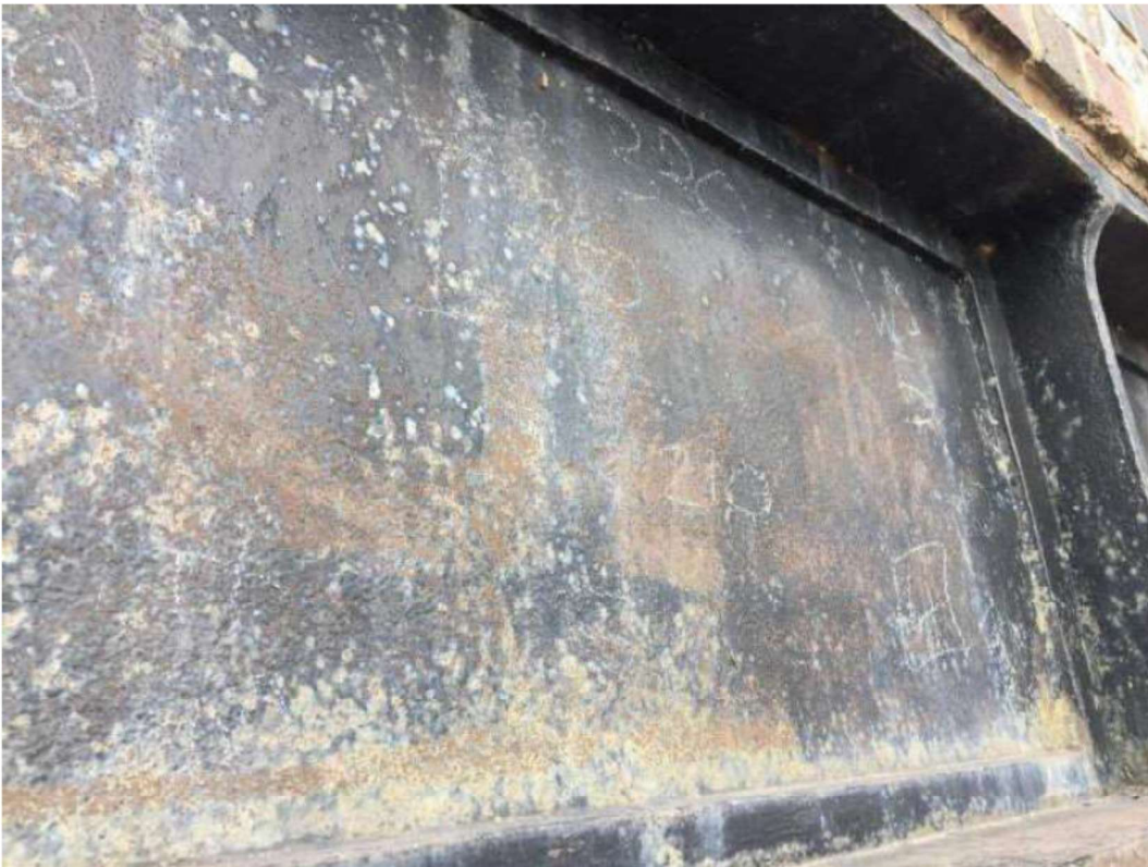
Photograph 22 - South edge girder outer face web print breakdown and surface corrosion
