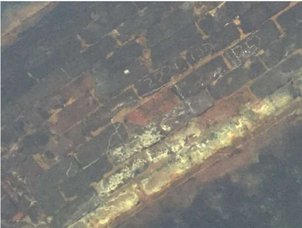
Photograph 29 - Isolated spalled bricks to all jack arches up to 30mm deep.
