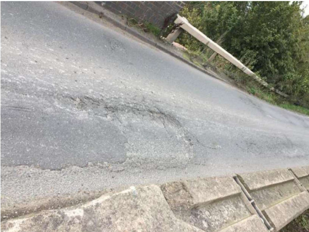
Photograph 20 - Typical carriageway condition – shows heavy crazing
