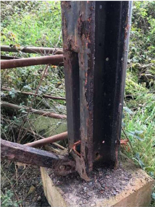
Photograph 39 - Edge north column prop channel (south east facing) - section loss of up to 4mm at base.
