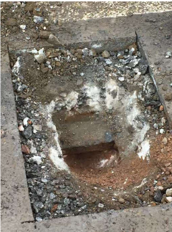
Photograph 42 – Trial pit 1 – Midspan, 1 st internal girder from north, exposing crown of 2 nd internal jack arch from north
