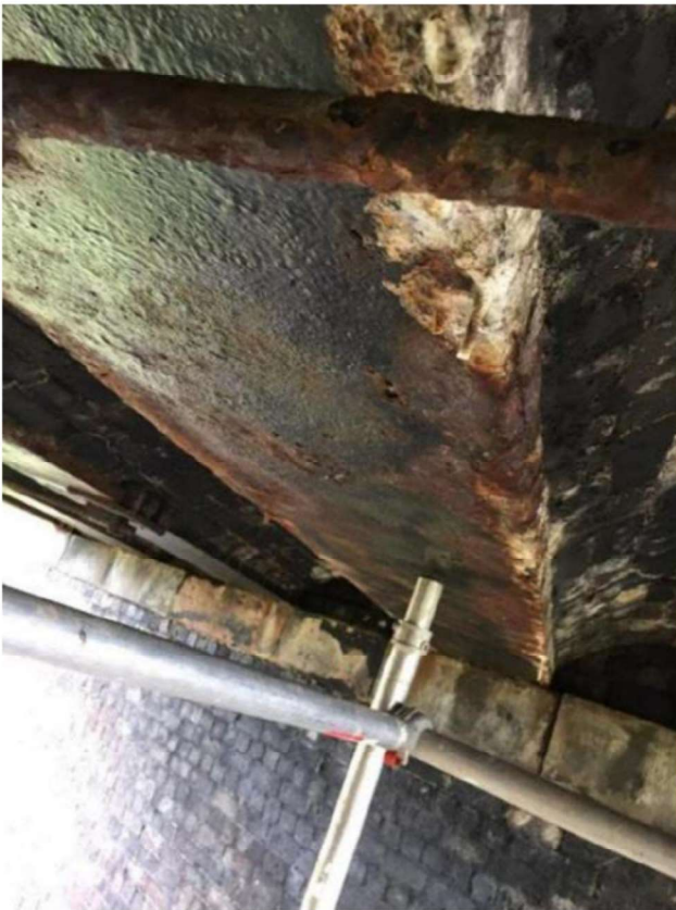
Photograph 27 - Typical 1mm deep corrosion to bottom flange of internal girders.
