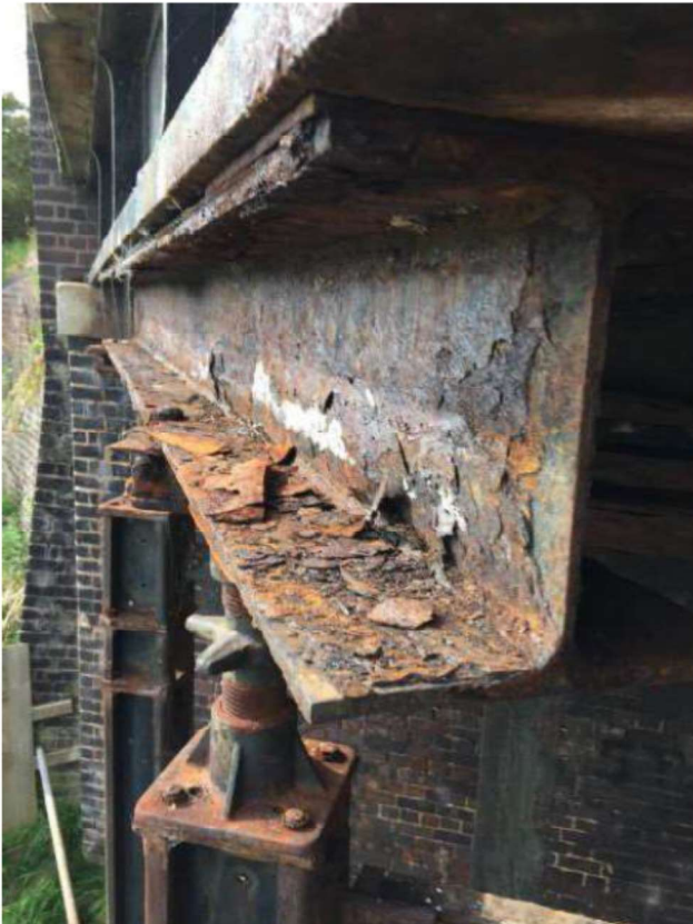
Photograph 36 - Delamination and corrosion to propping beams.
