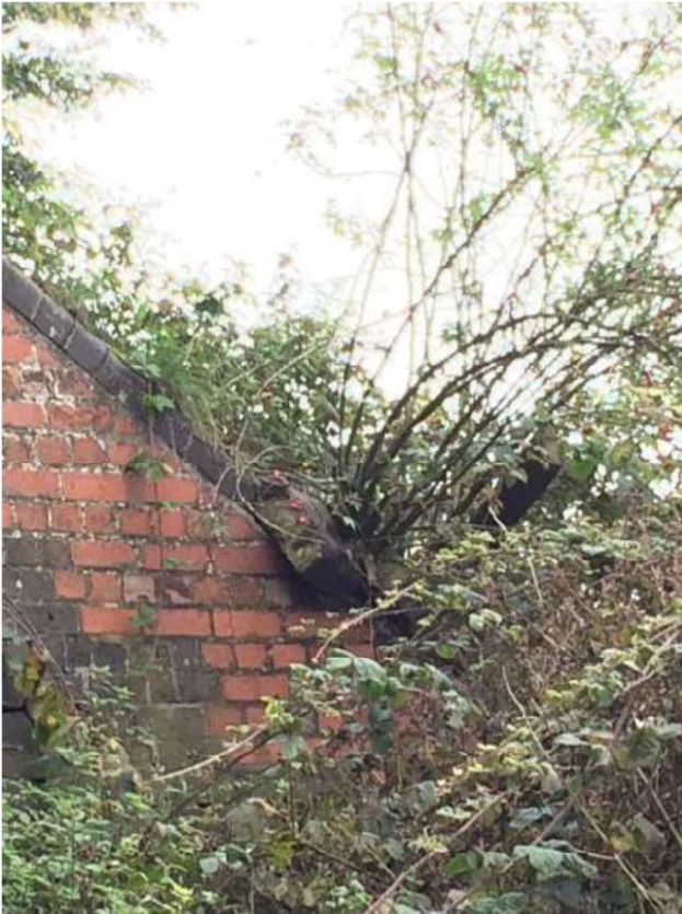
Photograph 33 - Dislocation to masonry of north west wingwall newel due to small tree growth
