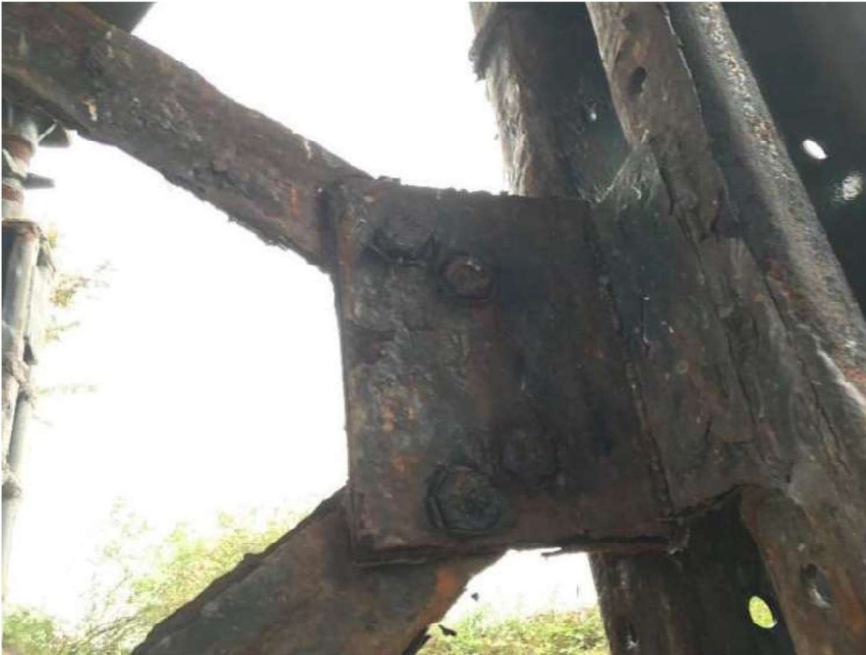
Photograph 41 - Delamination to bracing connection plates up to 2mm deep
