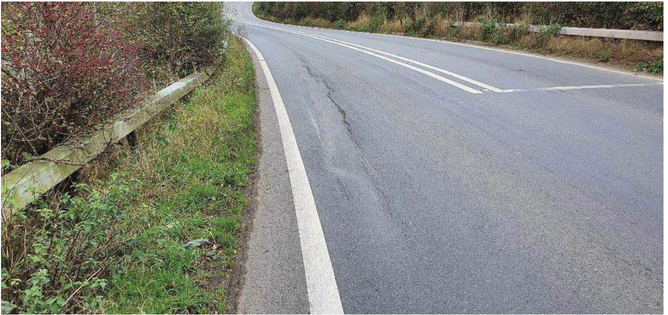
32. Settlement / crack in road surface to west
