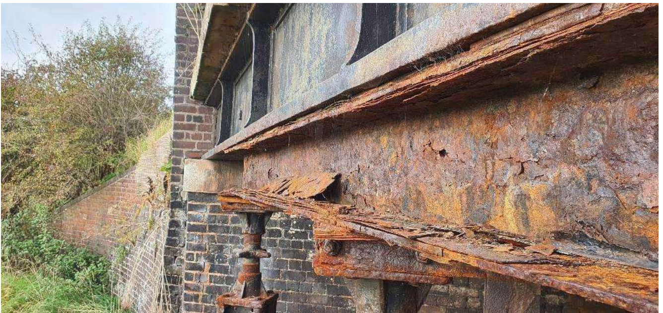
22. Typical condition of edge girders and propping beams
