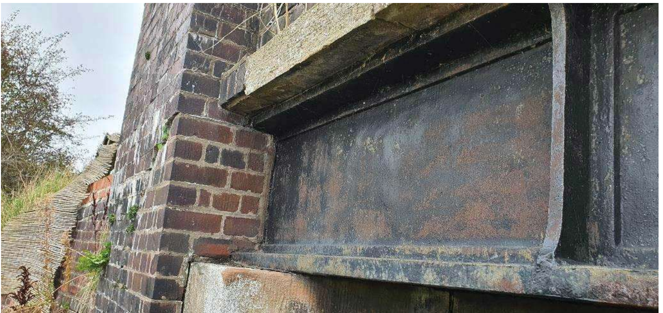
20. Typical condition of edge girders at support
