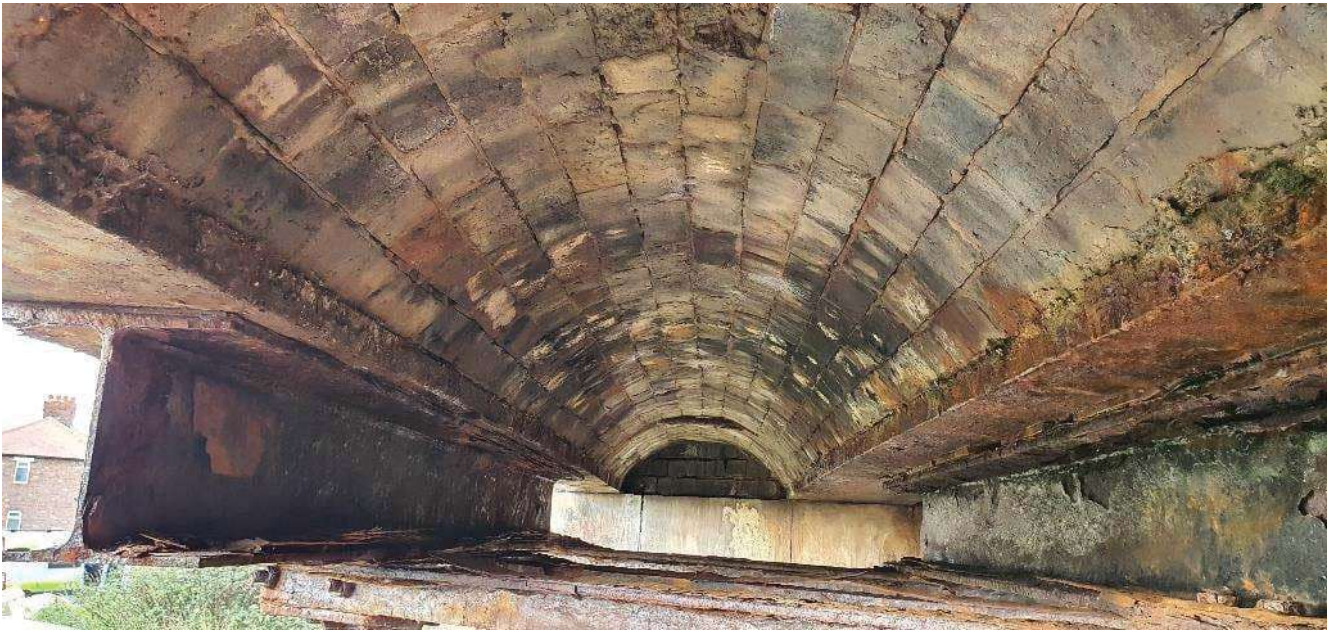
28. Typical edge jack arch bay condition
