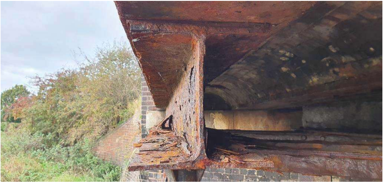
21. Typical condition of edge propping beams
