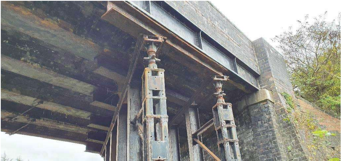
8. General view of soffit along propping
