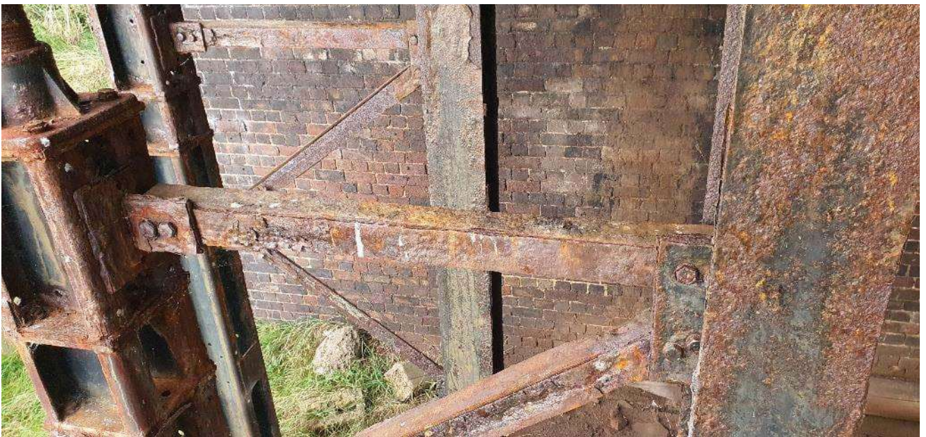
27. Typical bracing condition
