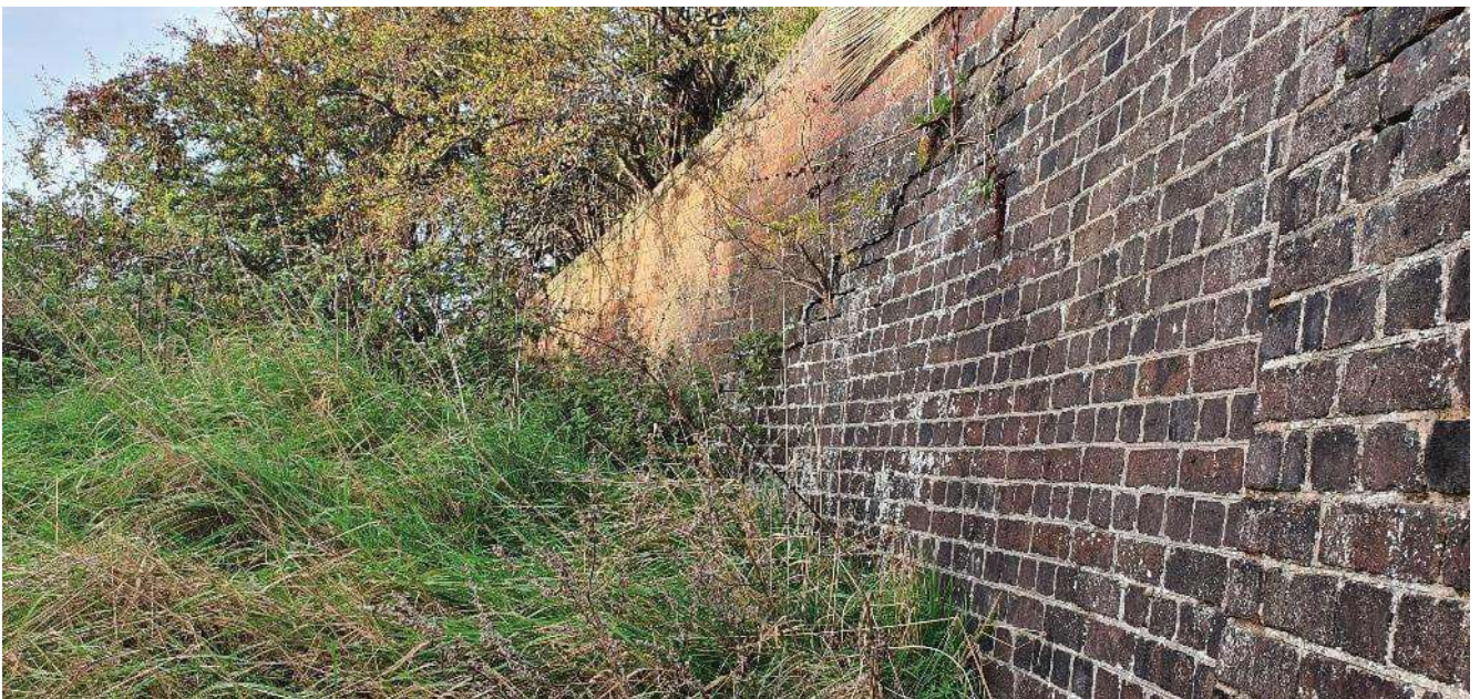
16. South west wingwall showing displacement to fracture
