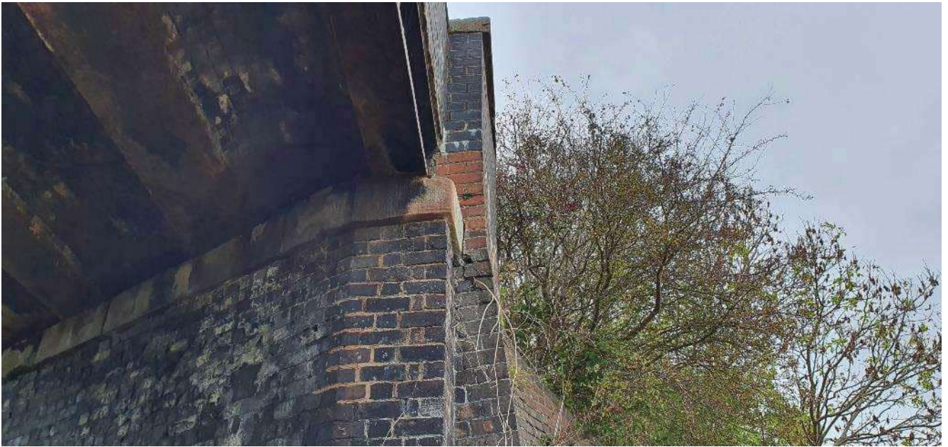
19. South east pilaster – showing fracture between pilaster and abutment
