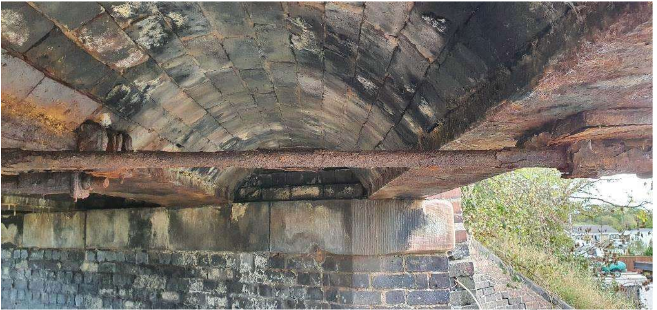
30. Typical condition of retro fitted ties
