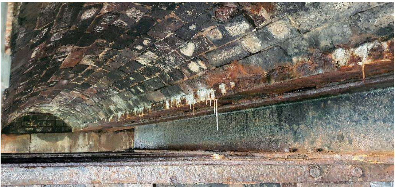
29. Typical internal jack arch bay condition
