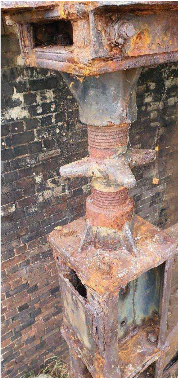
25. Condition of edge girder propping columns at top
