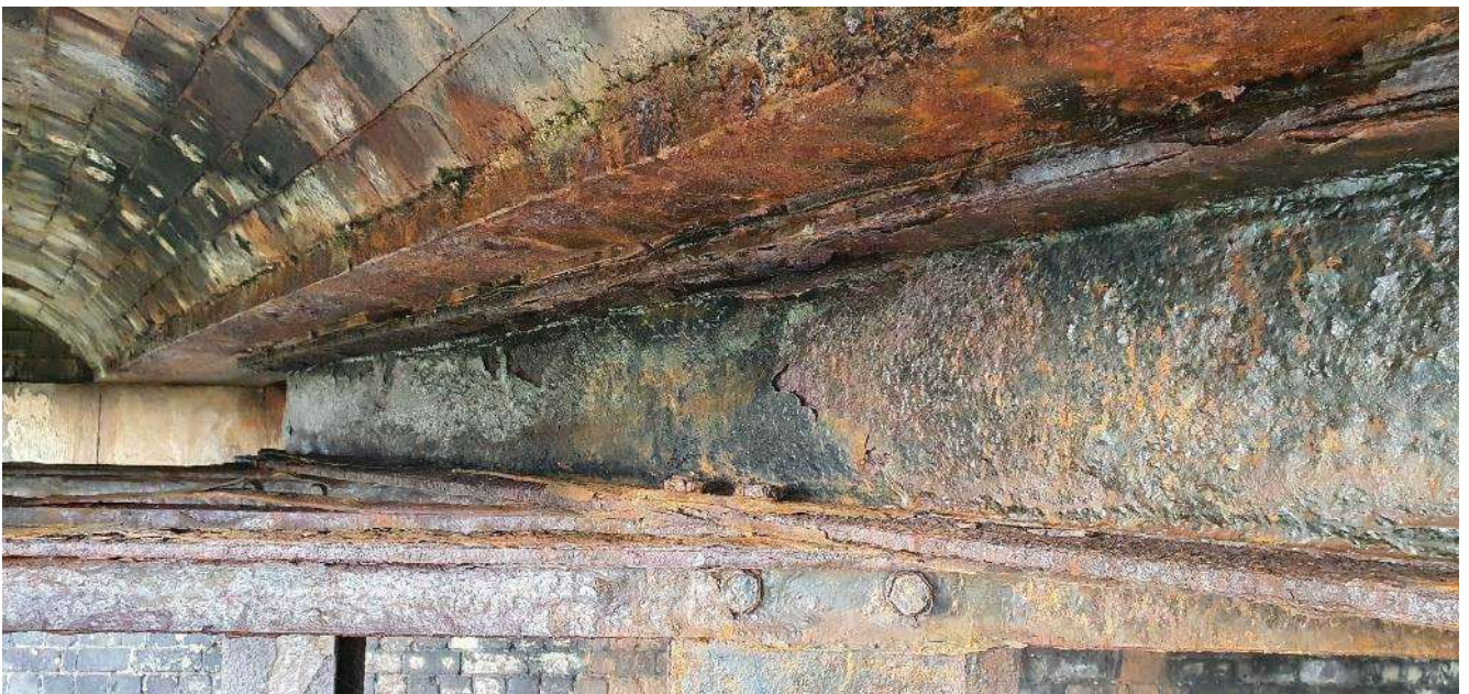
24. Typical condition of internal girders and propping beams
