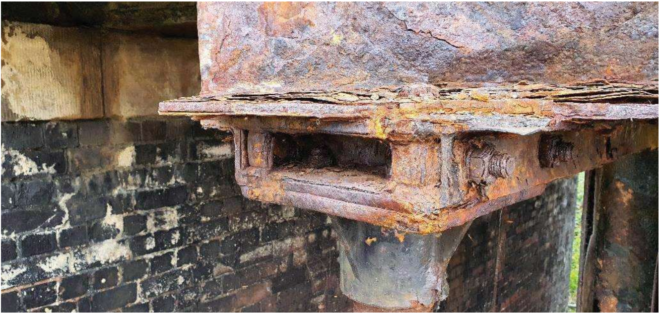
26. Condition of propping at interface between columns and beams
