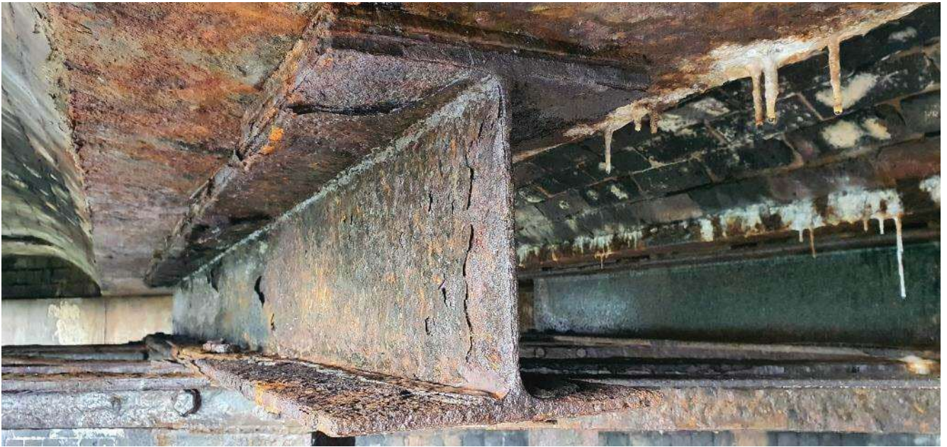
23. Typical condition of internal propping beams
