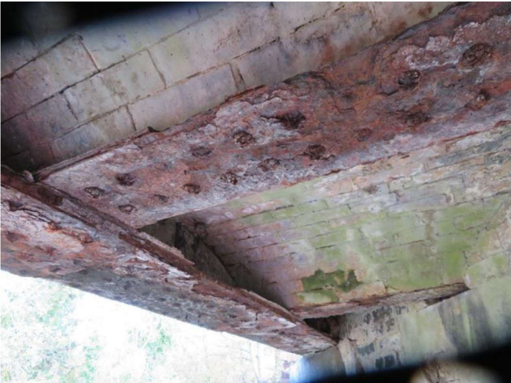
14. Condition of IG2
