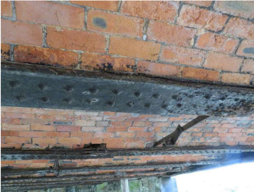
19. Typical condition at midspan (IG8 shown)
