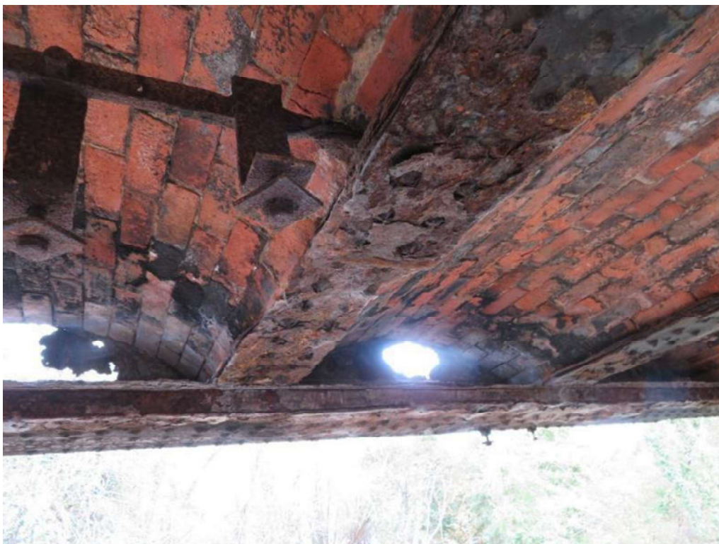
17. Typical condition of internal girders at support
