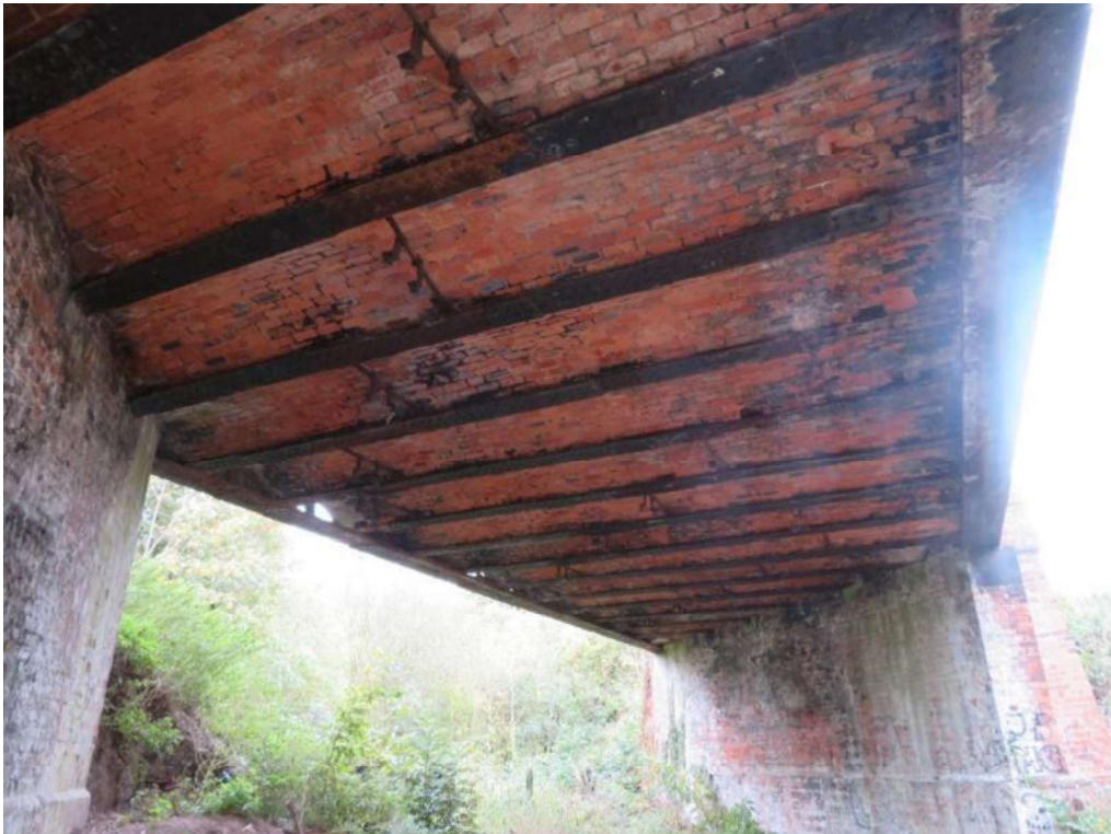
6. General soffit view looking west
