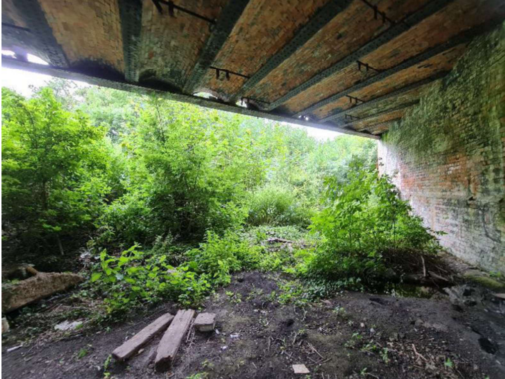
29. Formation looking south (2021 site visit)
