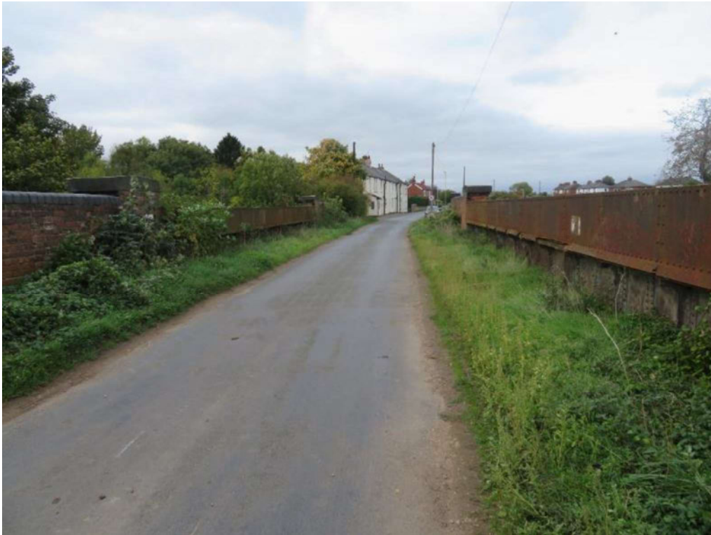
5. Road over structure looking west
