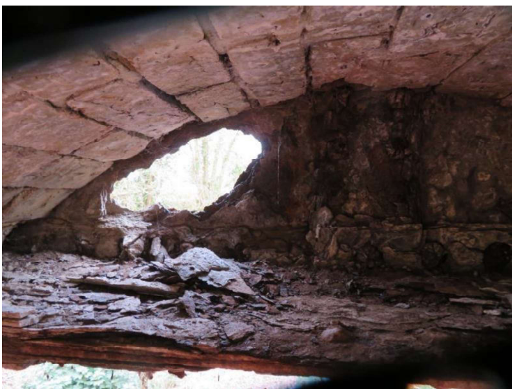
16. Typical edge girder condition below jack arch crowns
