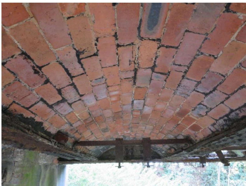
22. Typical jack arch condition
