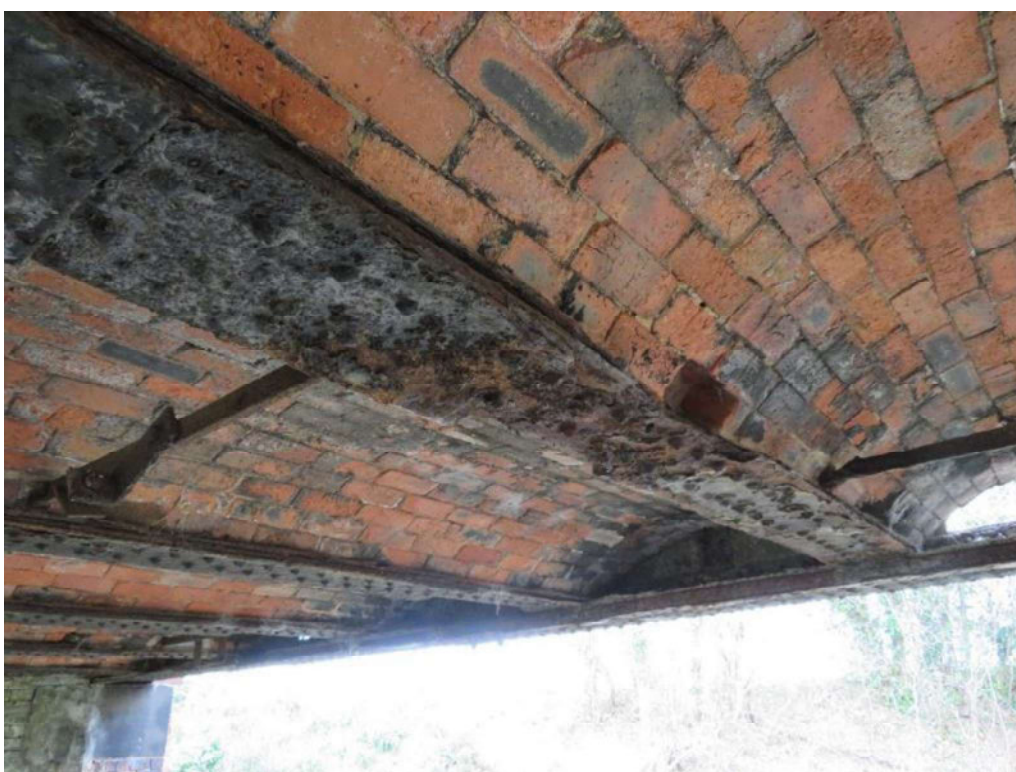
18. Typical condition of internal girders at third span (IG8 shown)
