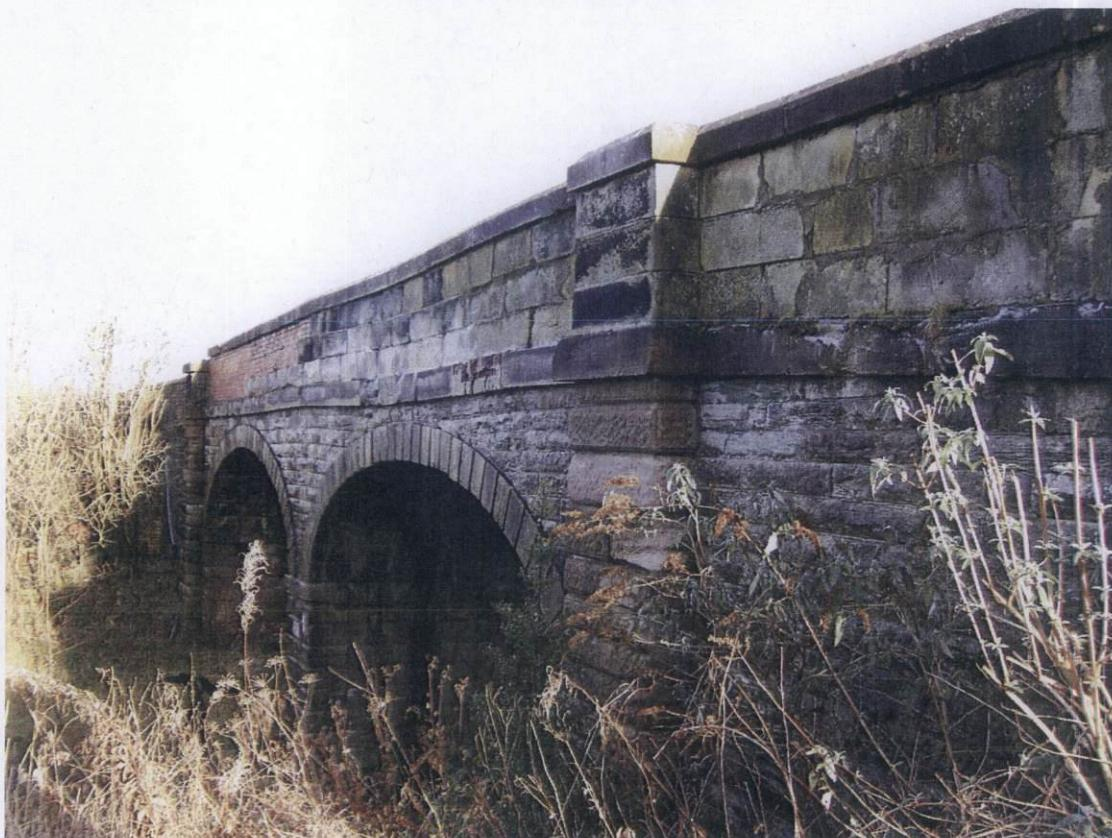
**Photograph 18:** West Spandrel and SW wingwall
