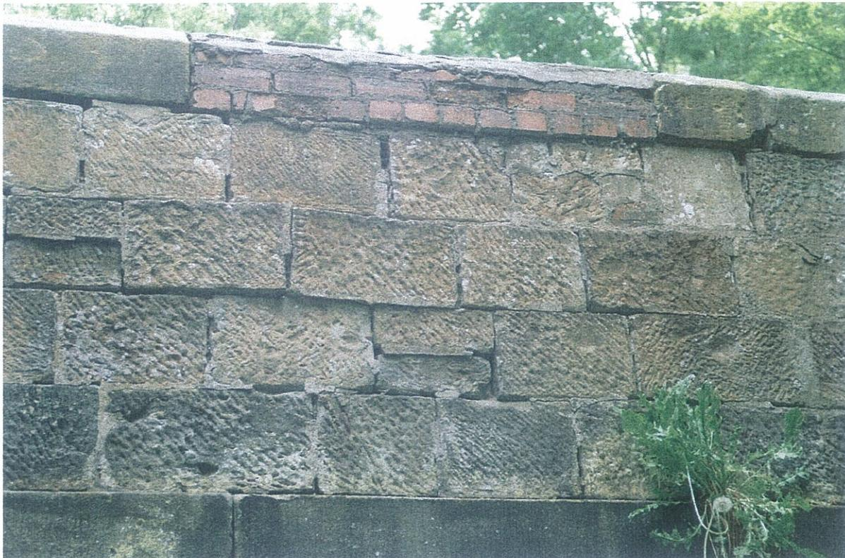
**Photograph 5 – Loose Masonry in Parapet**
