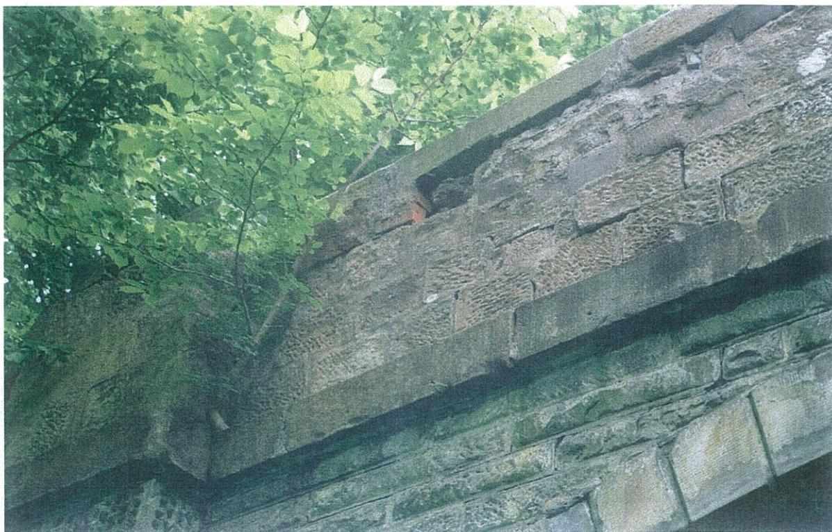
**Photograph 6 – Vegetation Growth and Loose/Missing Masonry in Parapet**
