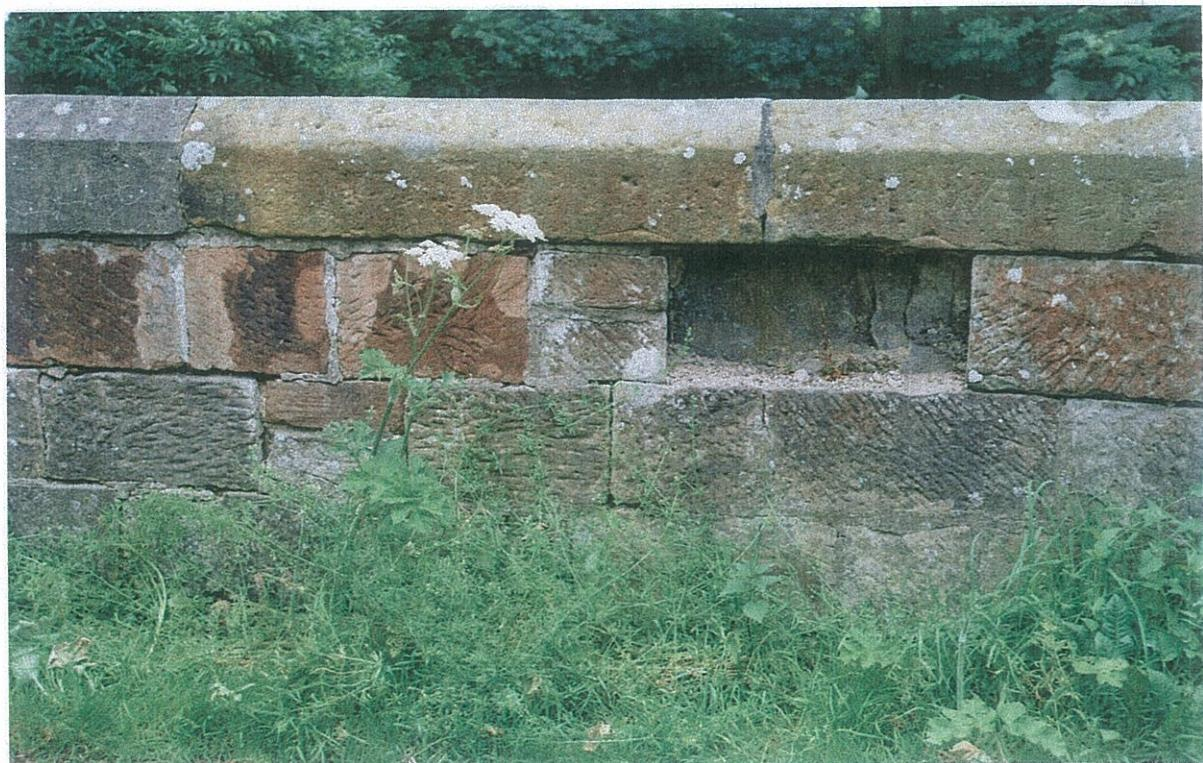
**Photograph 4 – Loose/Missing Masonry in Parapet**
