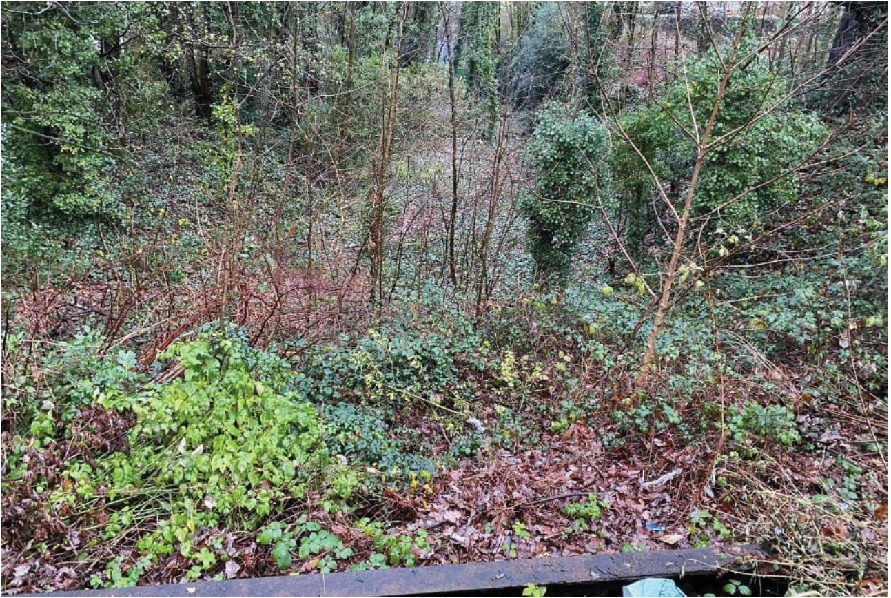
Photograph 29. Formation looking north
