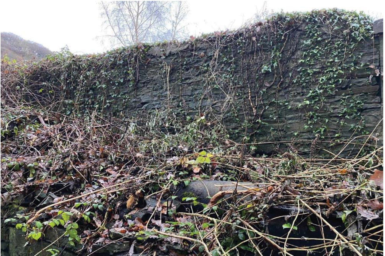
Photograph 11: North east wingwall
