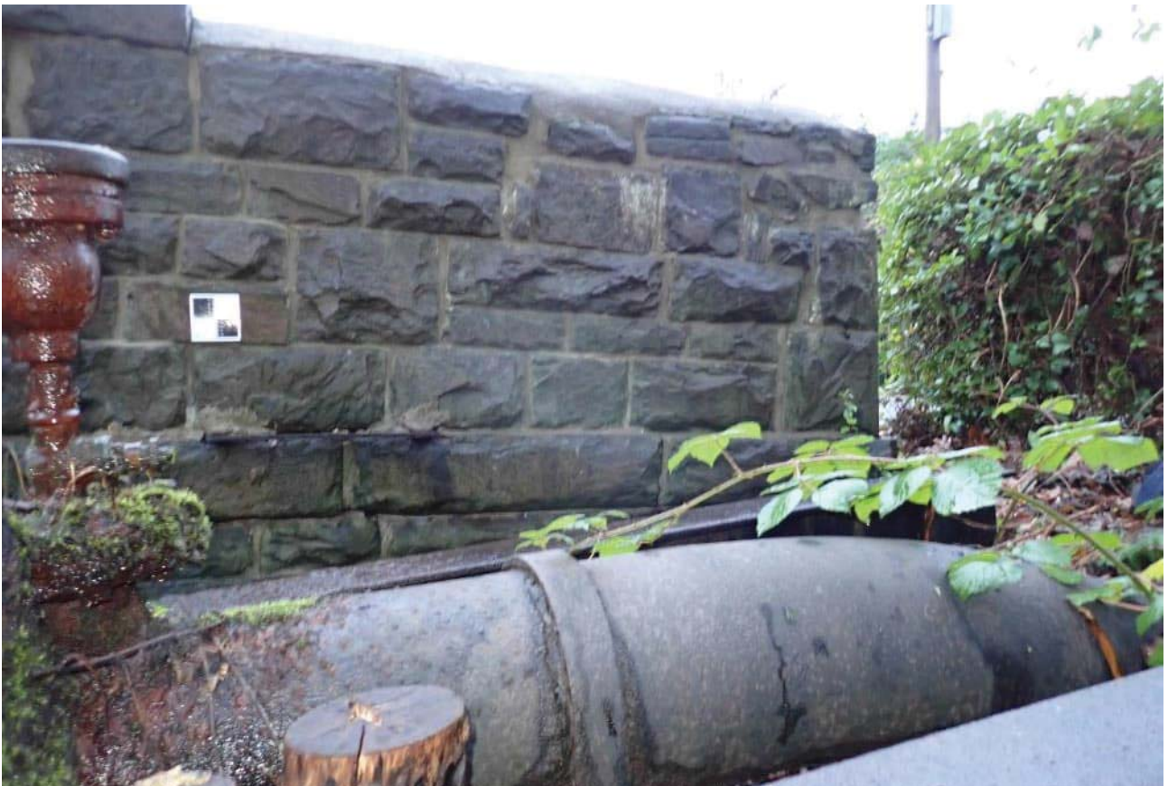
Photograph 12: North west wingwall
