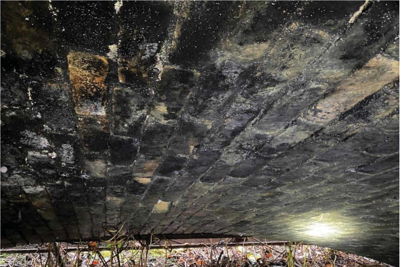
Photograph 7: Soffit at crown
