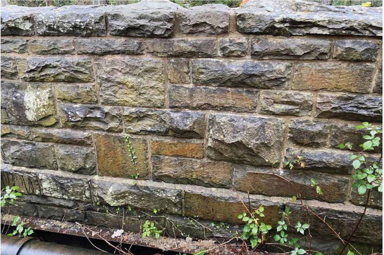
Photograph 13: South east wingwall
