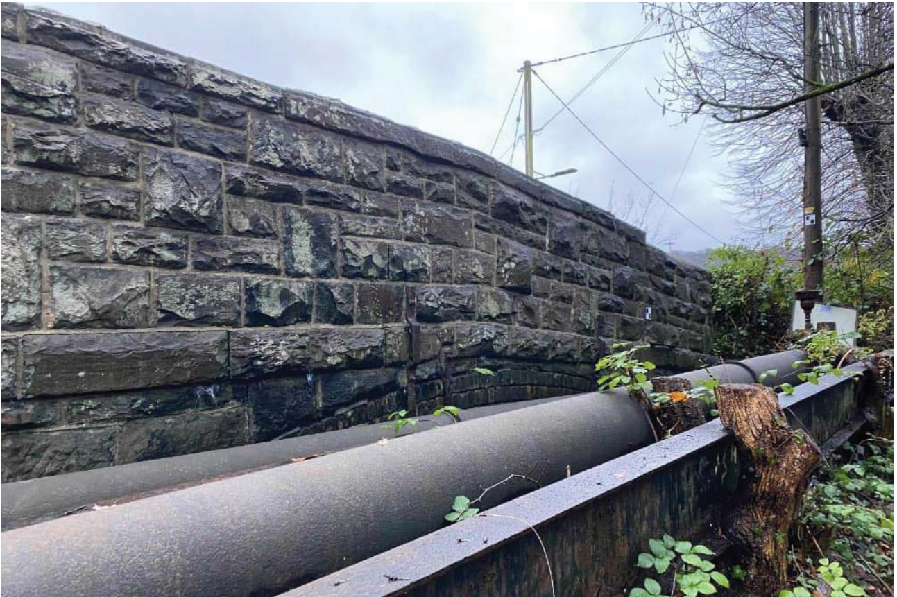
Photograph 15: North east spandrel
