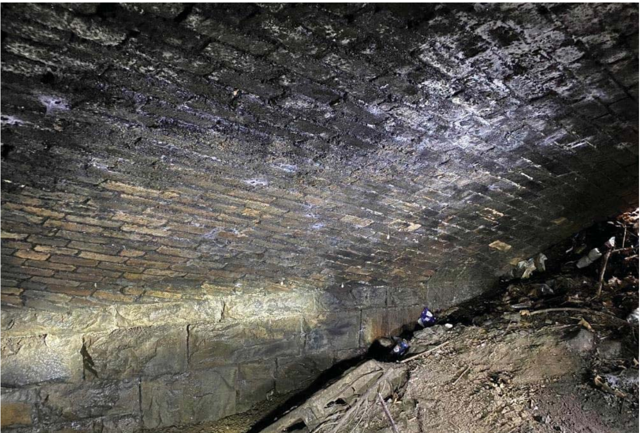
Photograph 8: Soffit at west haunch
