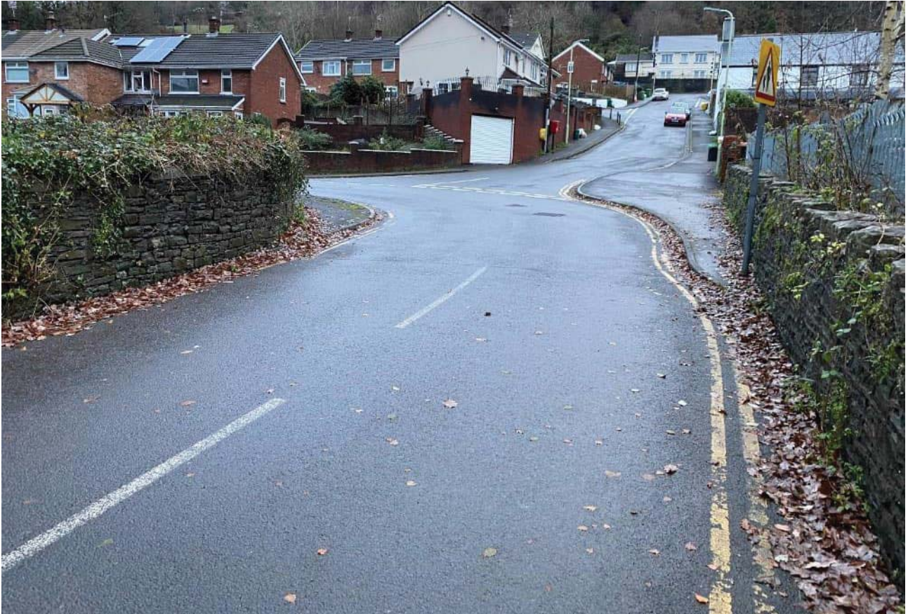
Photograph 3: Road approach looking east
