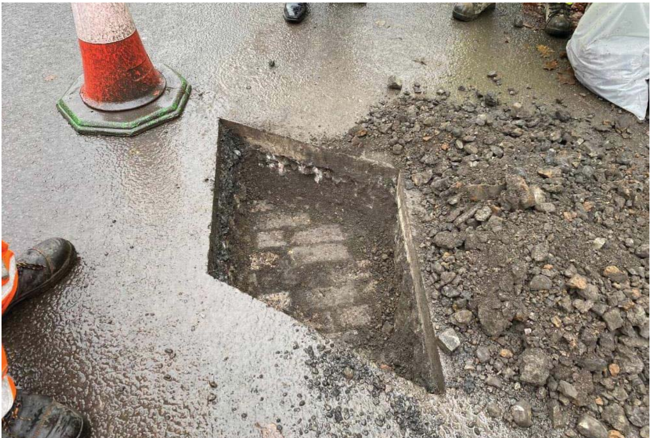
Photograph 32: Trial pit on top of the arch
