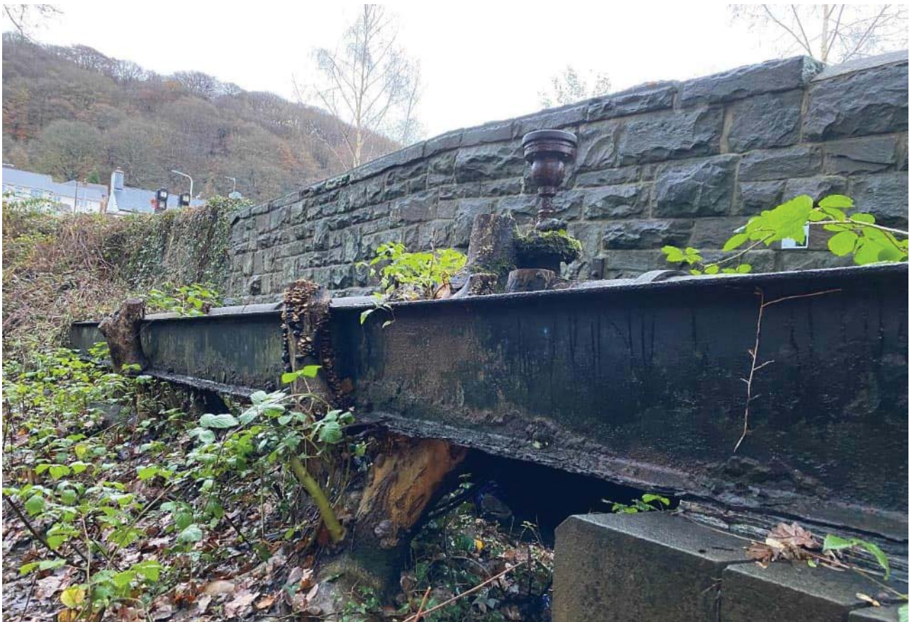
Photograph 16: North west spandrel
