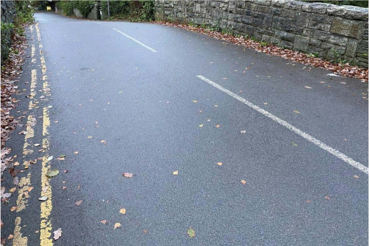
Photograph 5: Road over structure
