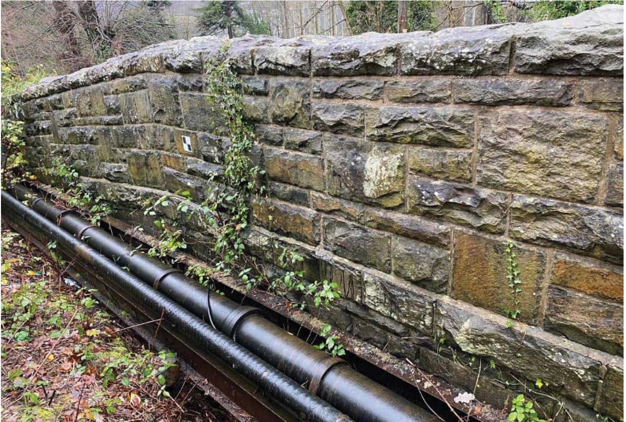
Photograph 17: South east spandrel
