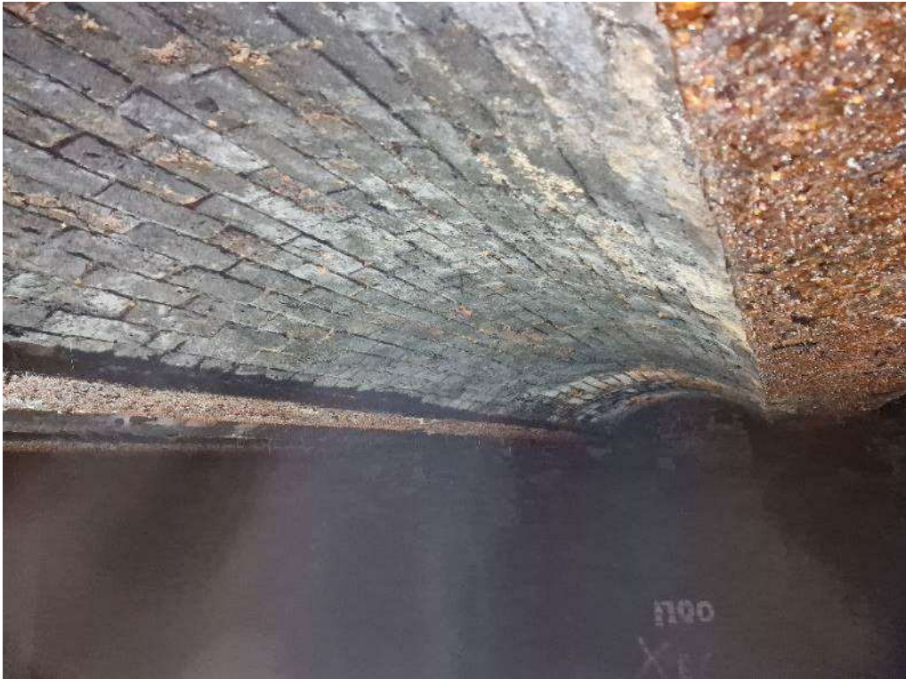
17. Typical jack arch condition (between girders 14 and 15 shown)
