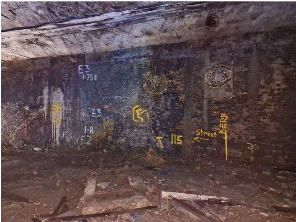
12. West sidewall beneath concrete encased steel girders
