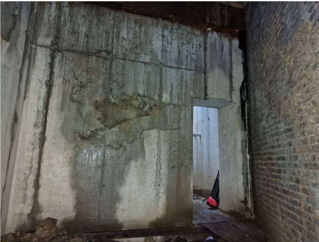
2. Blocked south portal (girder 41 visible at top of concrete wall)
