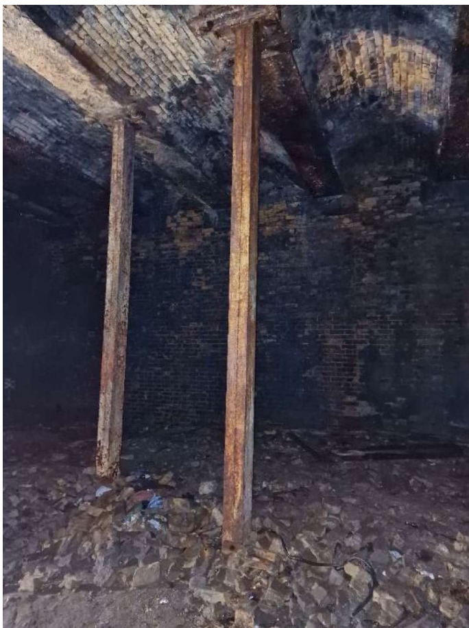
18. Propping columns (girder 11 right, girder 12 left)
