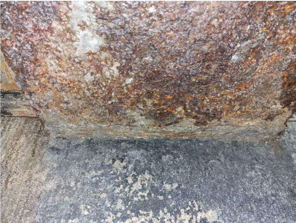
16. Typical cast iron girder condition (girder 16 in photo)
