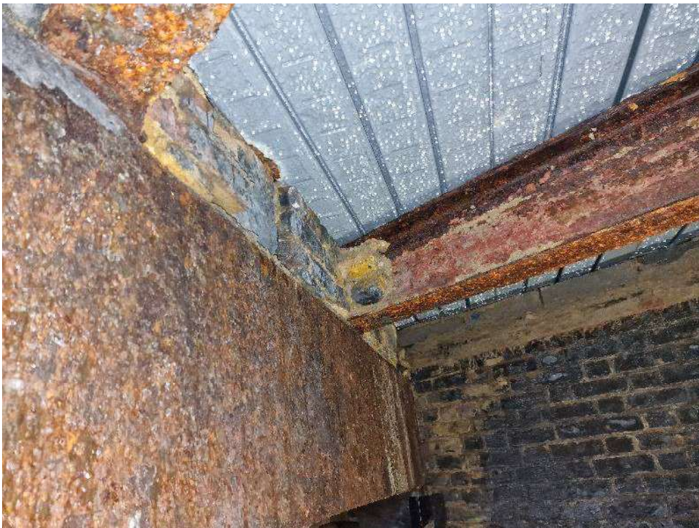
22. Typical RSJ and channel section condition (girder 41 on left of photo)
