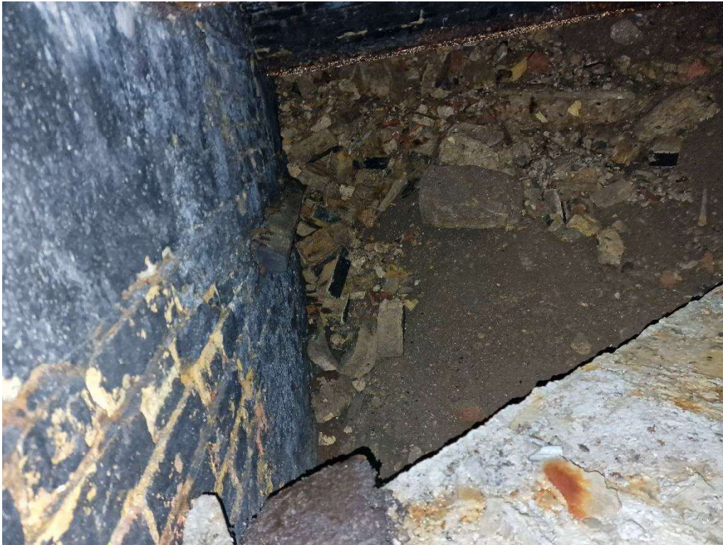
23. Backfill behind concrete retaining wall
