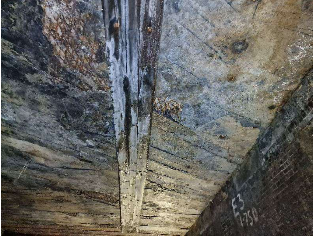
21. Spalling concrete along west thirdspan
