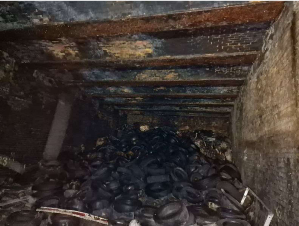
1. Blocked north portal (girders 1 to 7 visible)
