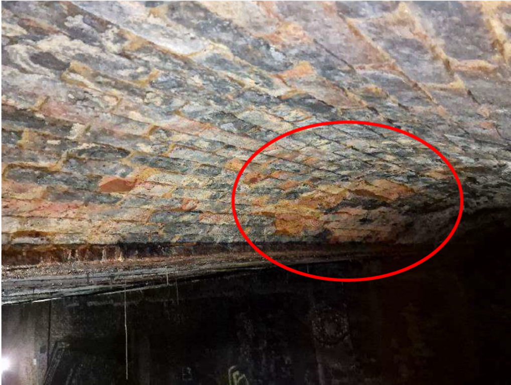
19. Spalling to jack arch between girders 18 and 19
