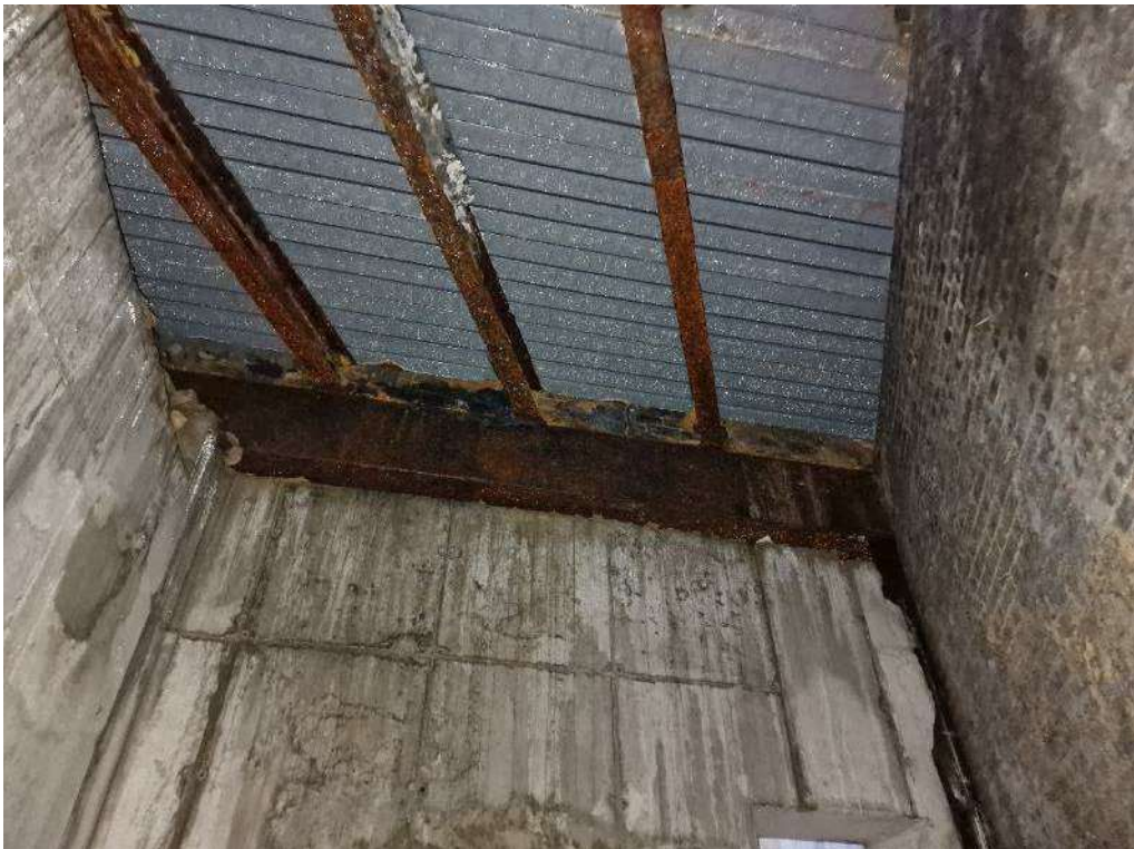
10. Visible section of south edge girder 41
