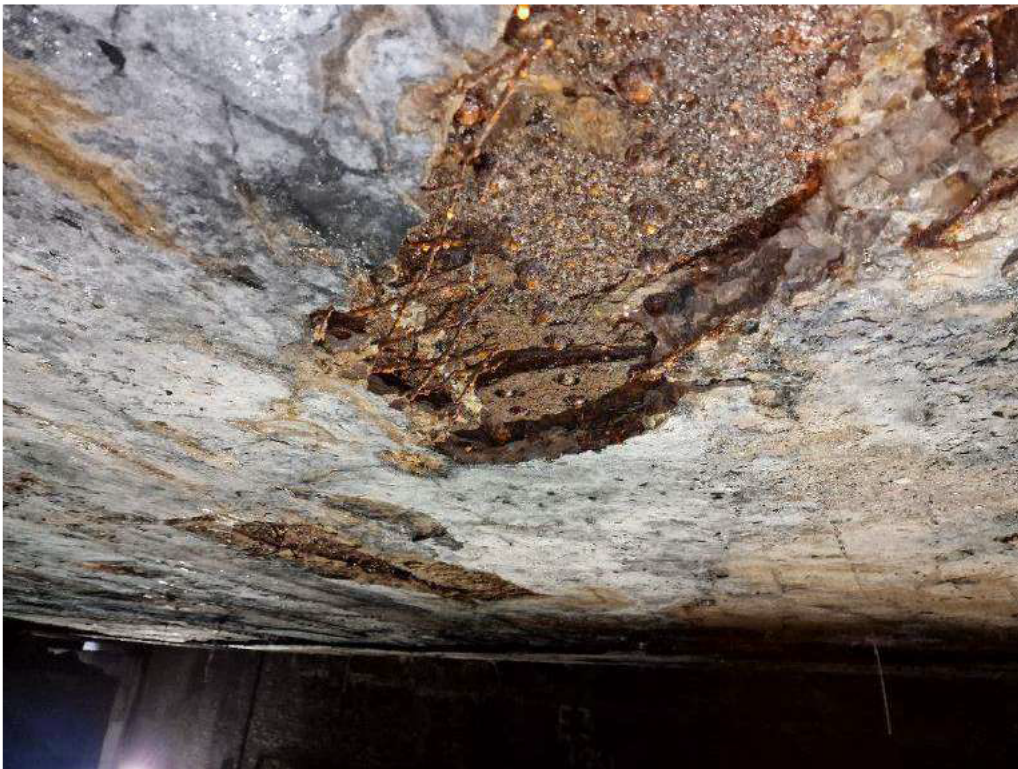
20. Spalled concrete and corrosion at east end of girders 25 and 26
