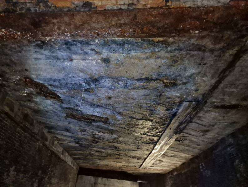
7. General soffit view of concrete encased steel girder section (girder 19 at top of photo)
