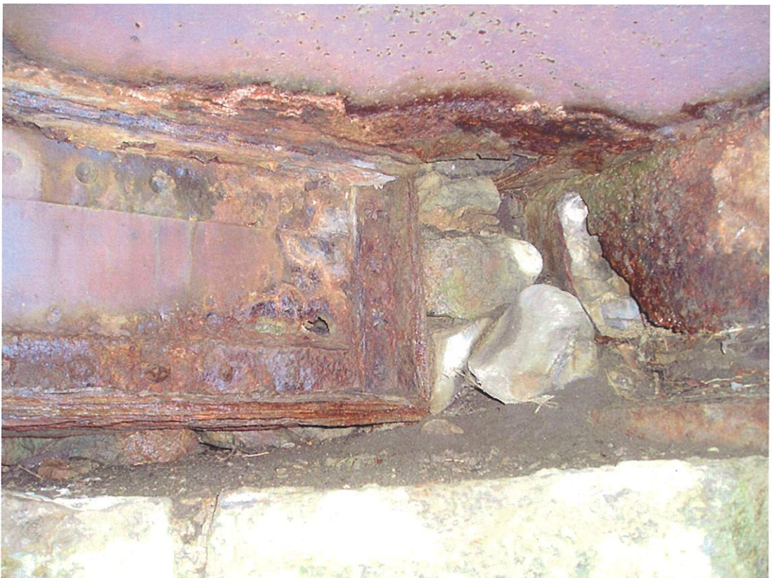
Holes in main and cross girders in south west corner of structure
