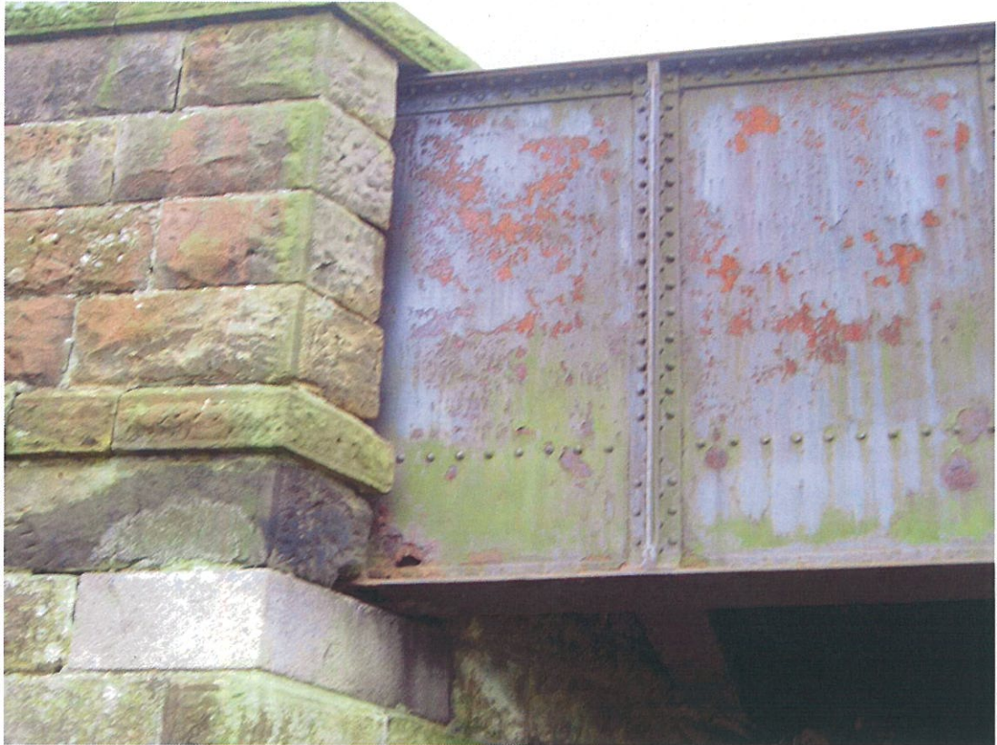
Hole in east main girder
