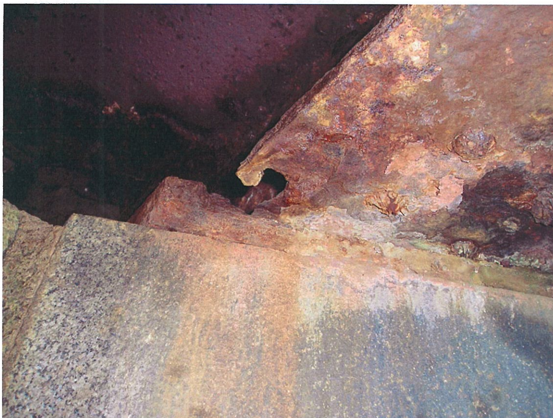
Corrosion to bottom flange of west main girder adjacent to south abutment
