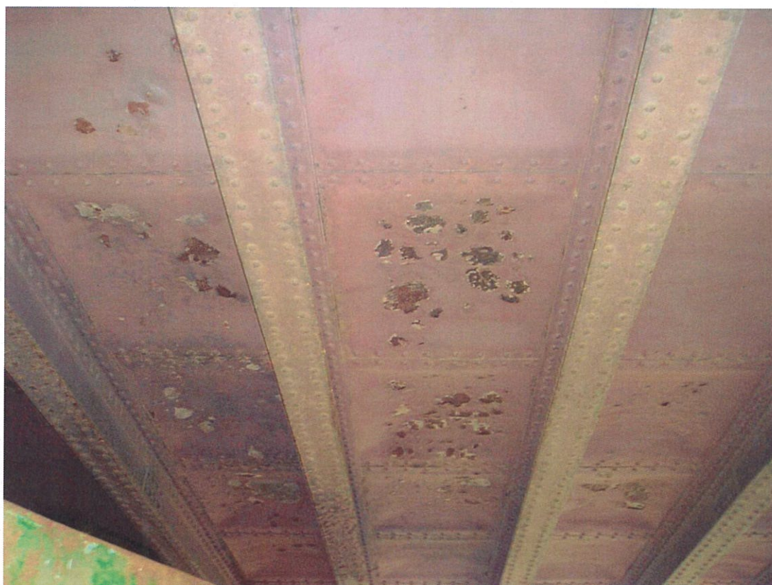
Deck plates and cross girders
