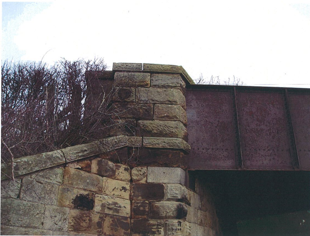
Open joints in north west pilaster
