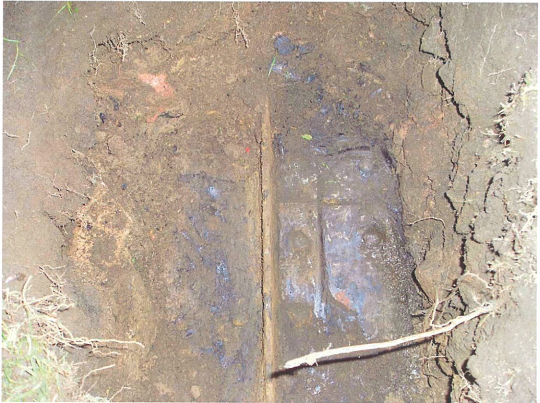
Trial pit exposing deck plate and tee section
