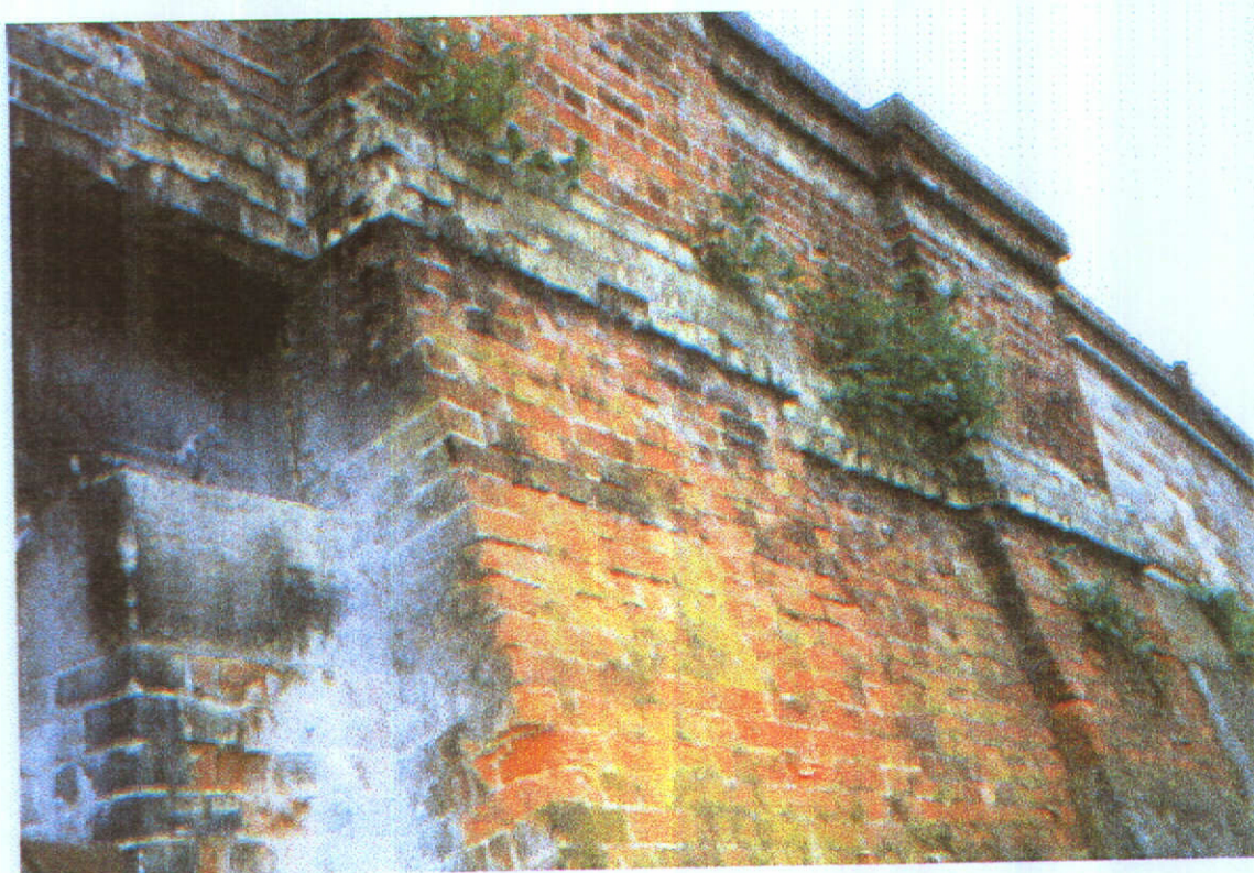
Photograph 6 - North east wing wall showing spalling and vegetation growth
