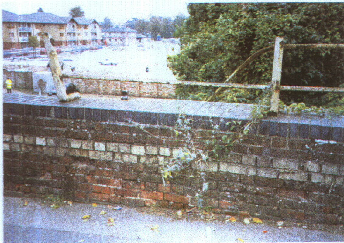
Photograph 11 – Damage to steel post and rail at south end of east parapet
