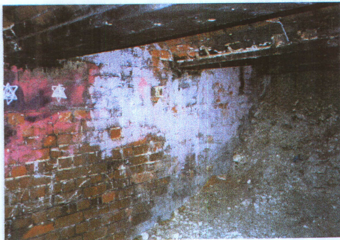
Photograph 14 – View of east abutment showing backfill covering west elevation.
