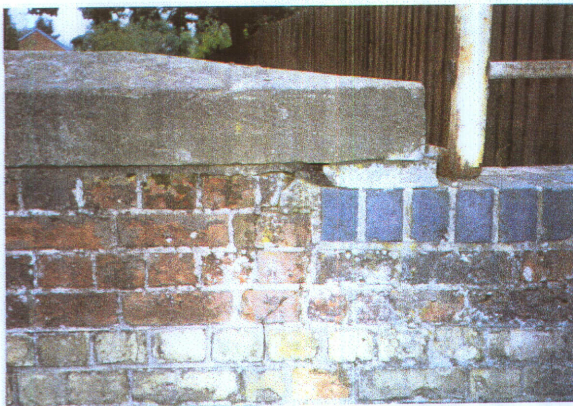
Photograph 13 – Displaced coping stone to south pilaster
