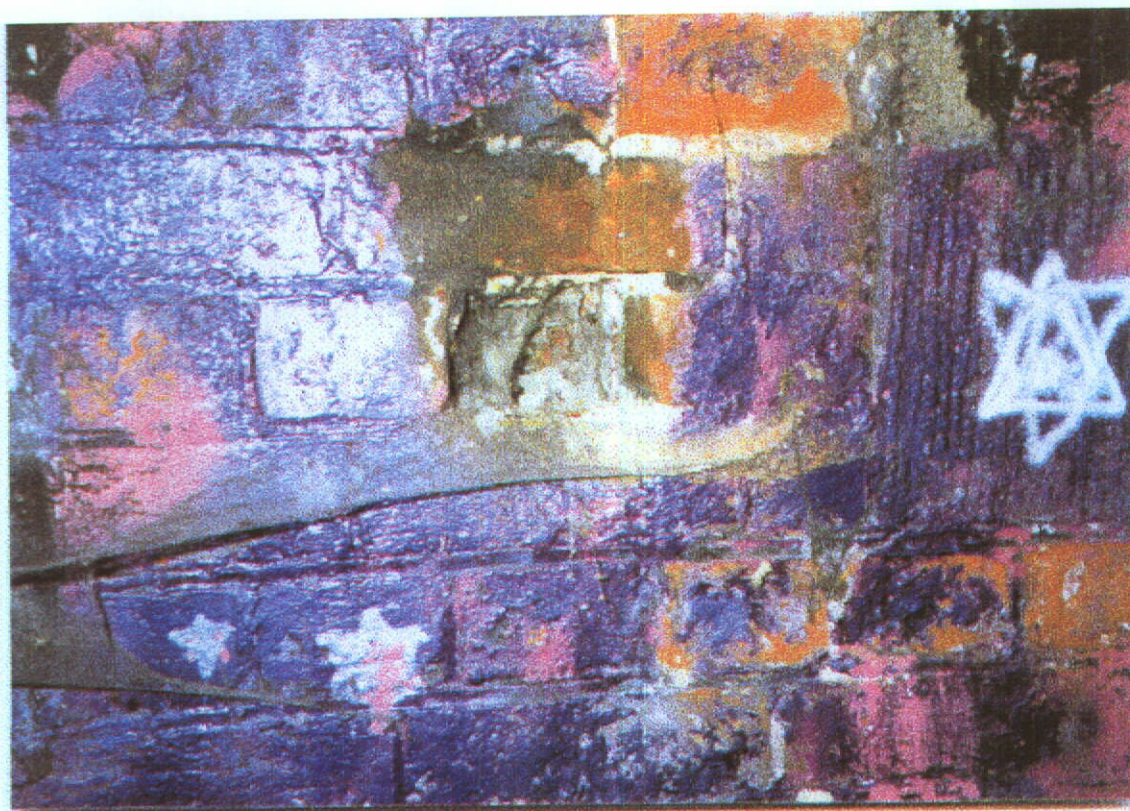
Photograph 15 – Missing brick, typical to the east abutment
