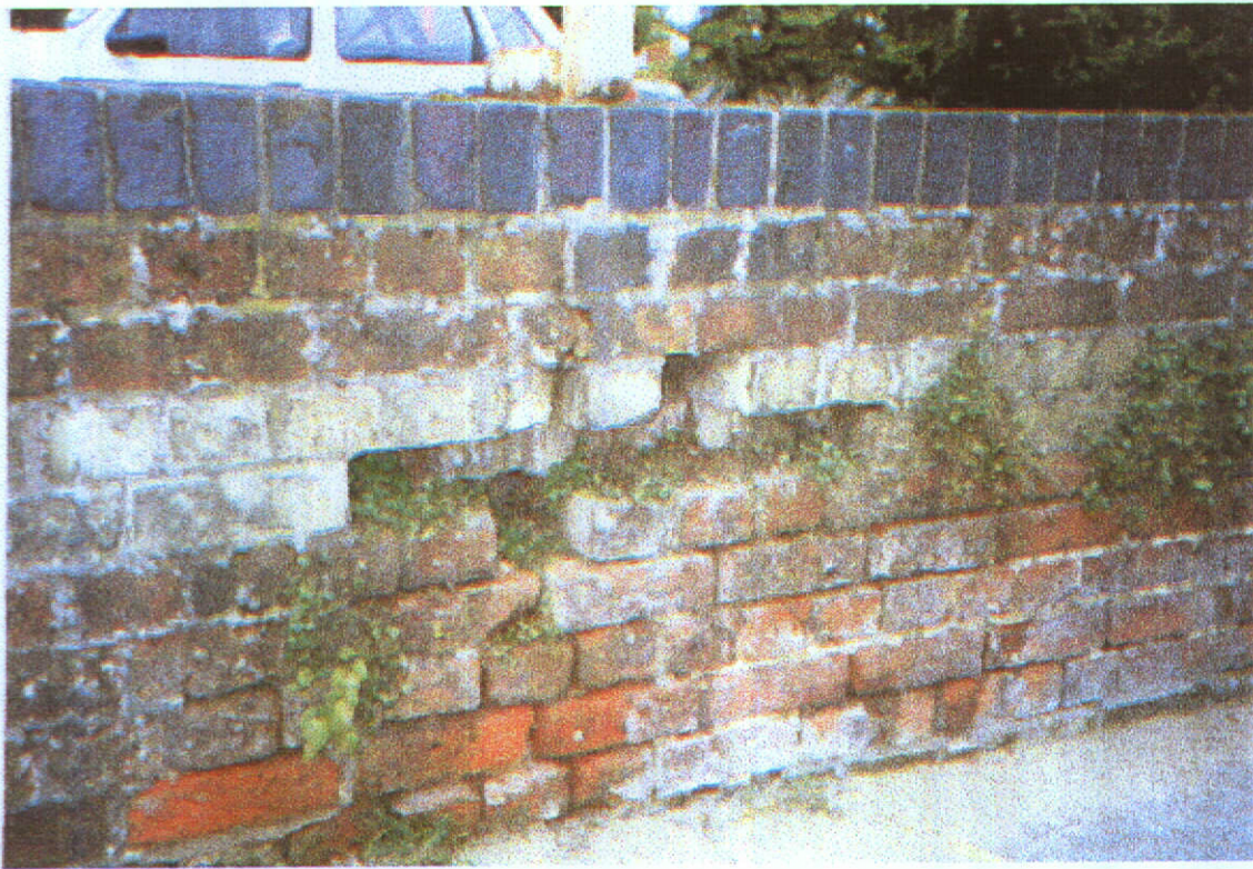
Photograph 7 – Missing brickwork from west parapet
