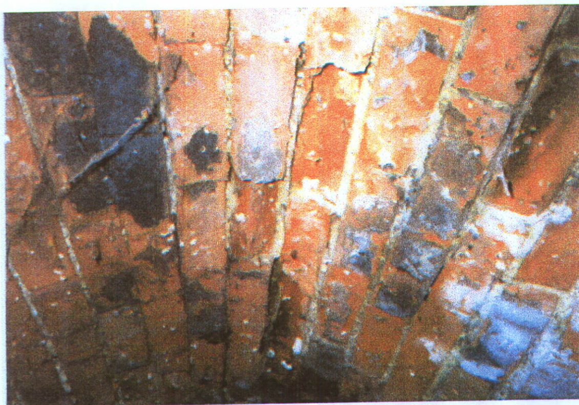
Photograph 5 – Typical spalling brickwork on jack arch soffit
