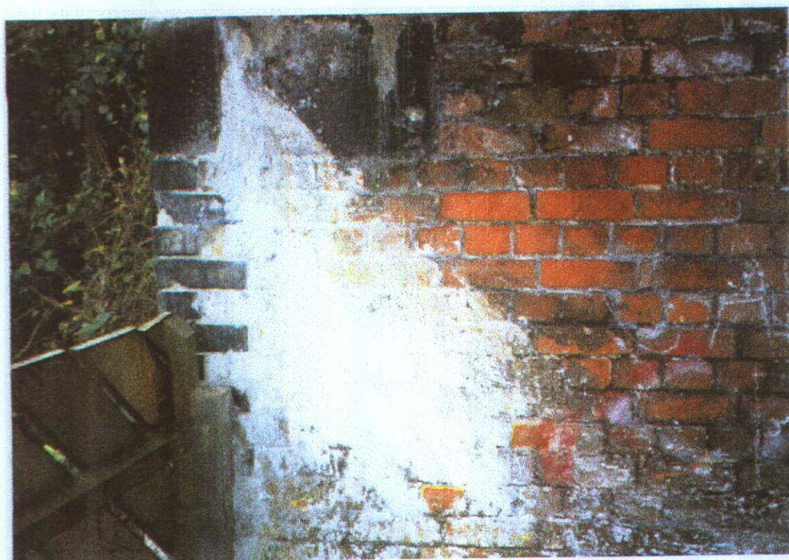
Photograph 12 – Leach staining on south abutment
