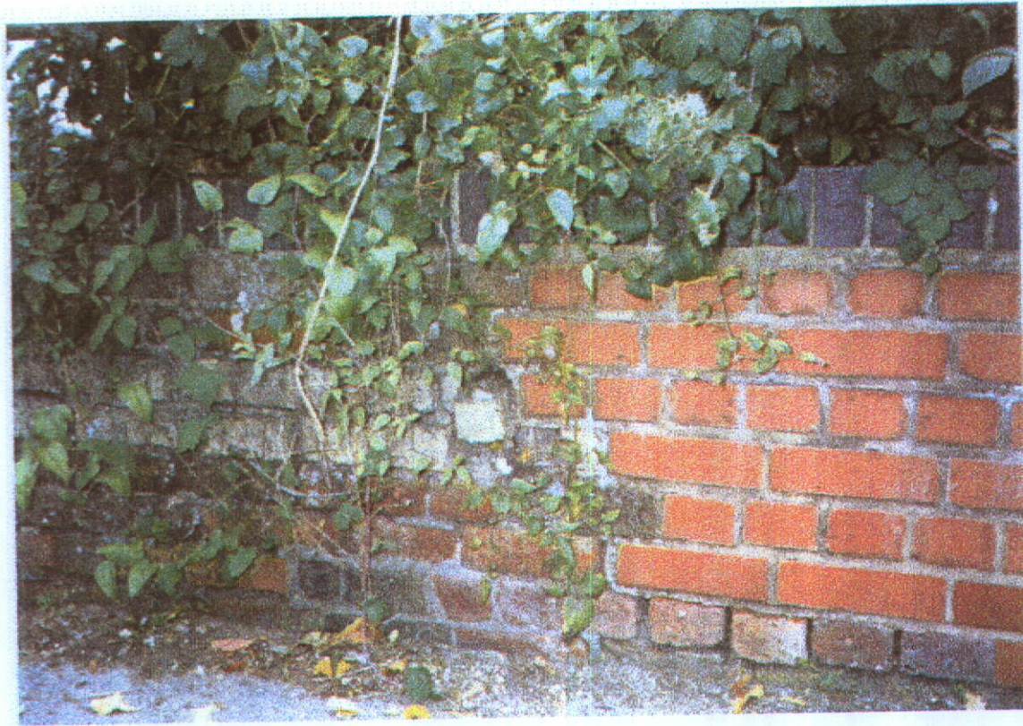
Photograph 9 – Loss of brickwork from joint between old and new brickwork at the south end of the east parapet
